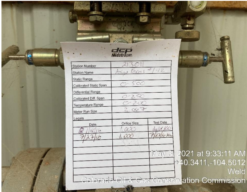
Photo #3 Meter not calibrated annually
