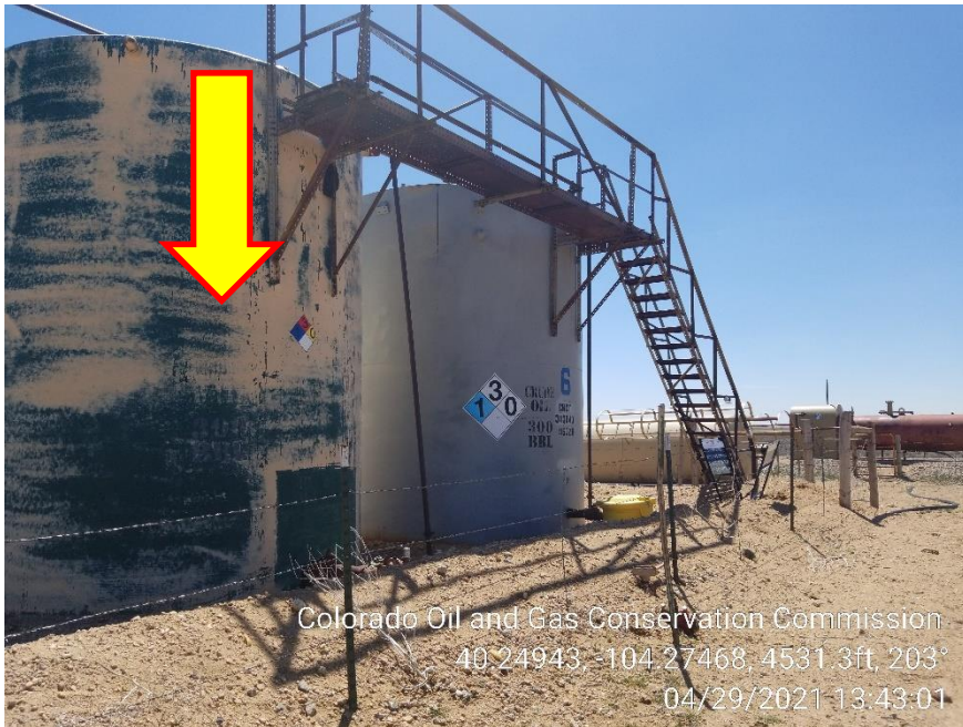
Photo 1 – Tank Battery – H2O Tank missing Content and Capacity
