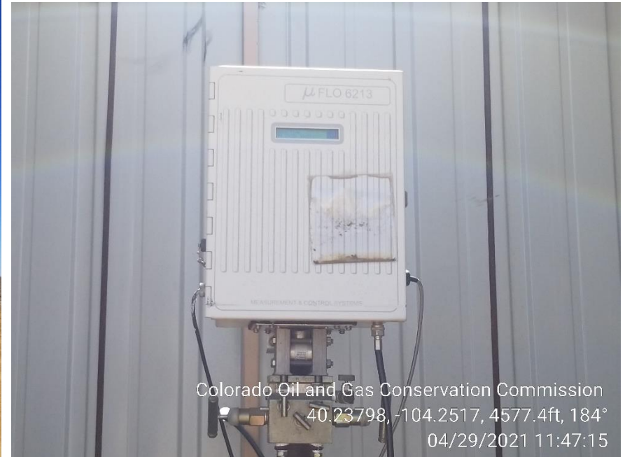
Photo 4 – Gas Meter Calibration Card NOT Present
