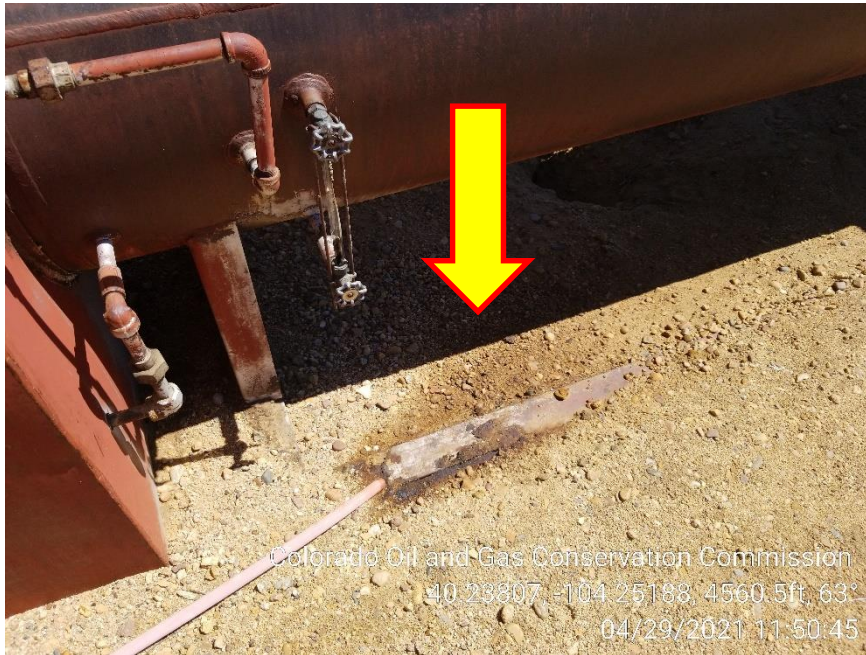
Photo 7 – Stained Soil at Separator
