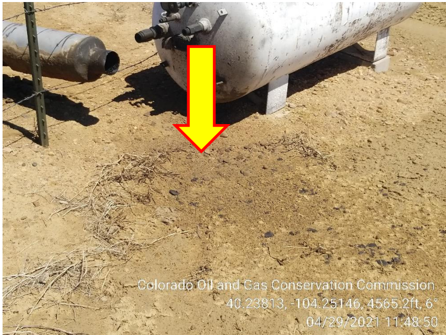
Photo 9 – Stained Soil at Gas Engine Exhaust
