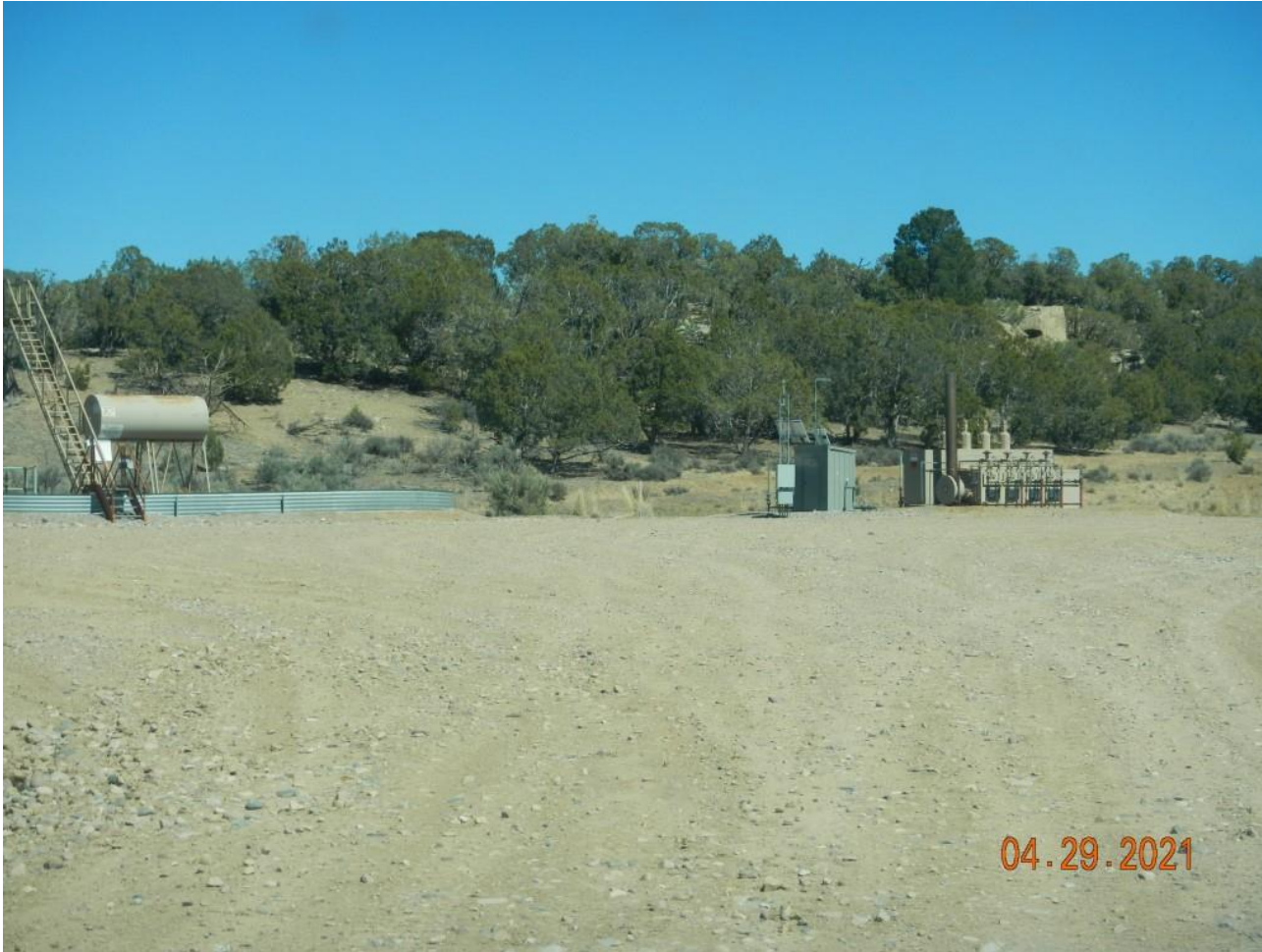
Photo#1: Overview of Location from entry.
