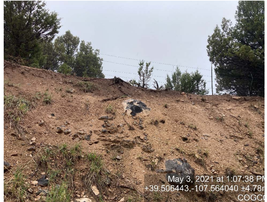
Lack of stabilization/erosion
