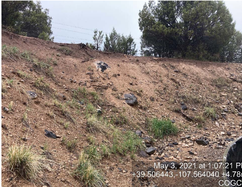
Lack of stabilization/erosion
