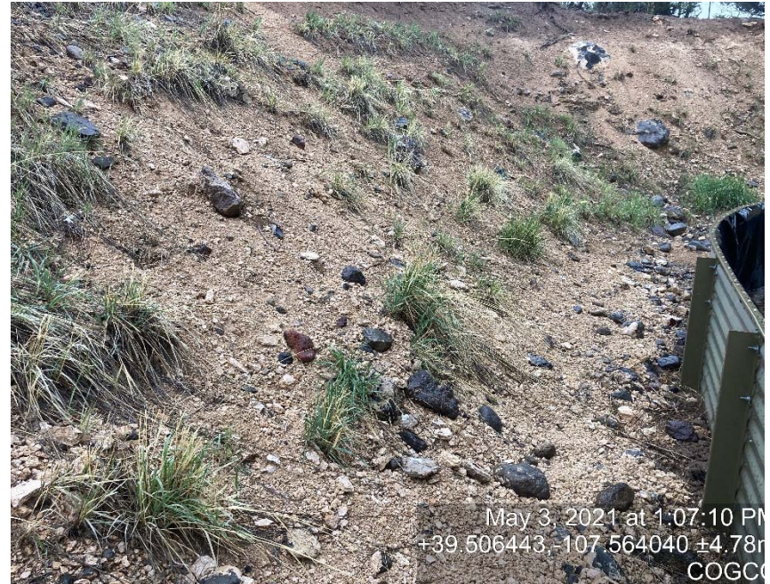
Lack of stabilization/erosion
