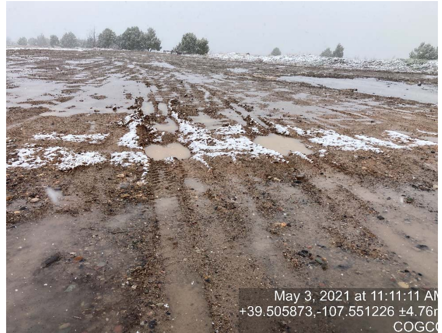
Lack of stabilization/compaction
