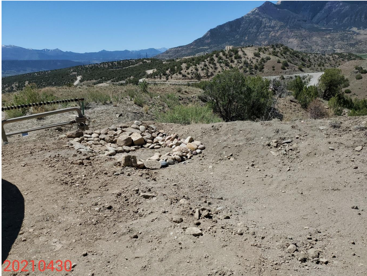
Photo 3: Photo taken from the south end of the Location, facing southwest. Photo shows Operator has installed a sediment trap and slope drain; It is unclear at time of inspection if control measures are adequate or sufficient for the site's conditions.
