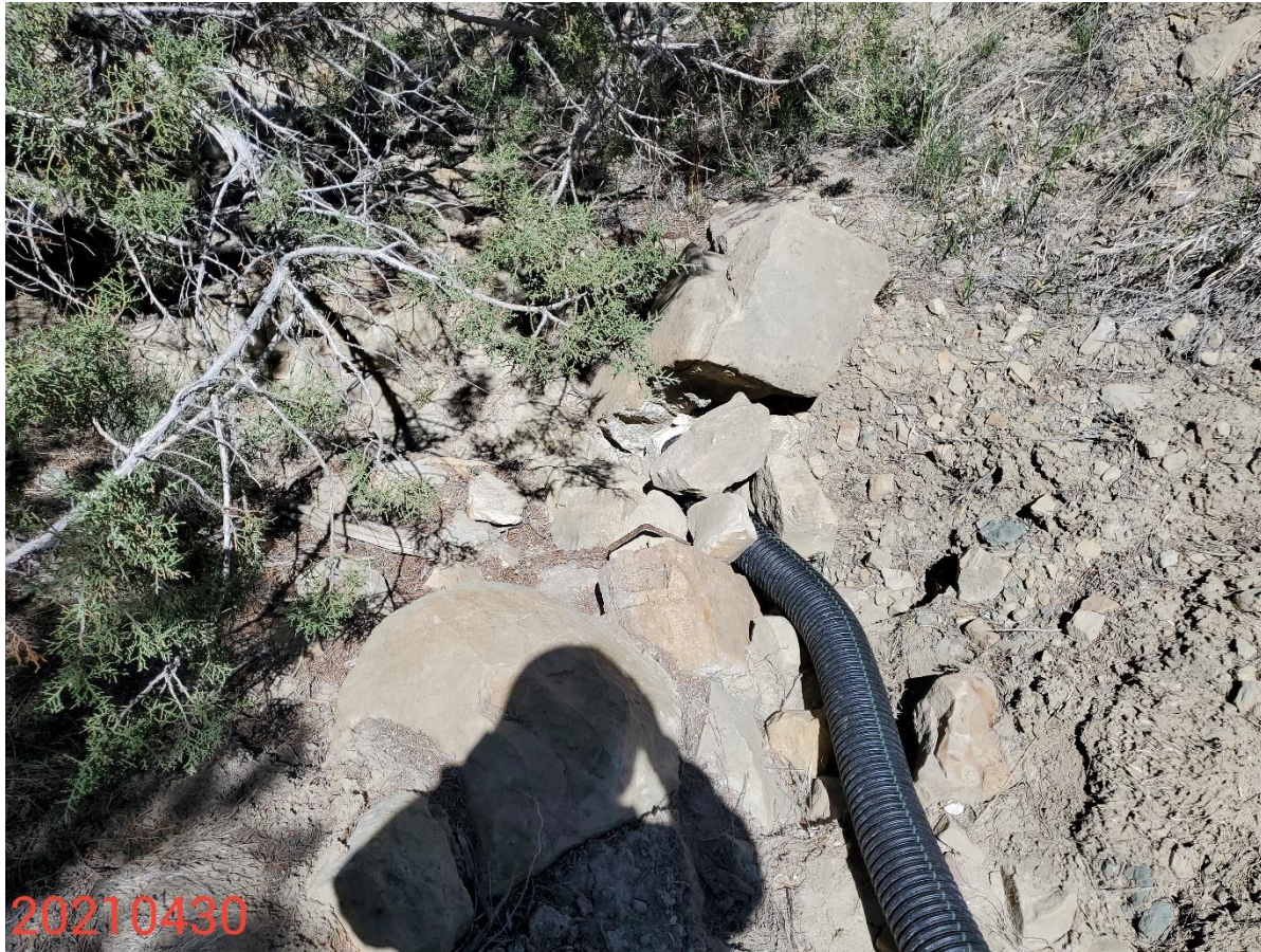
Photo 5 Photo of the slope drain outlet. See comments under photo 3.
