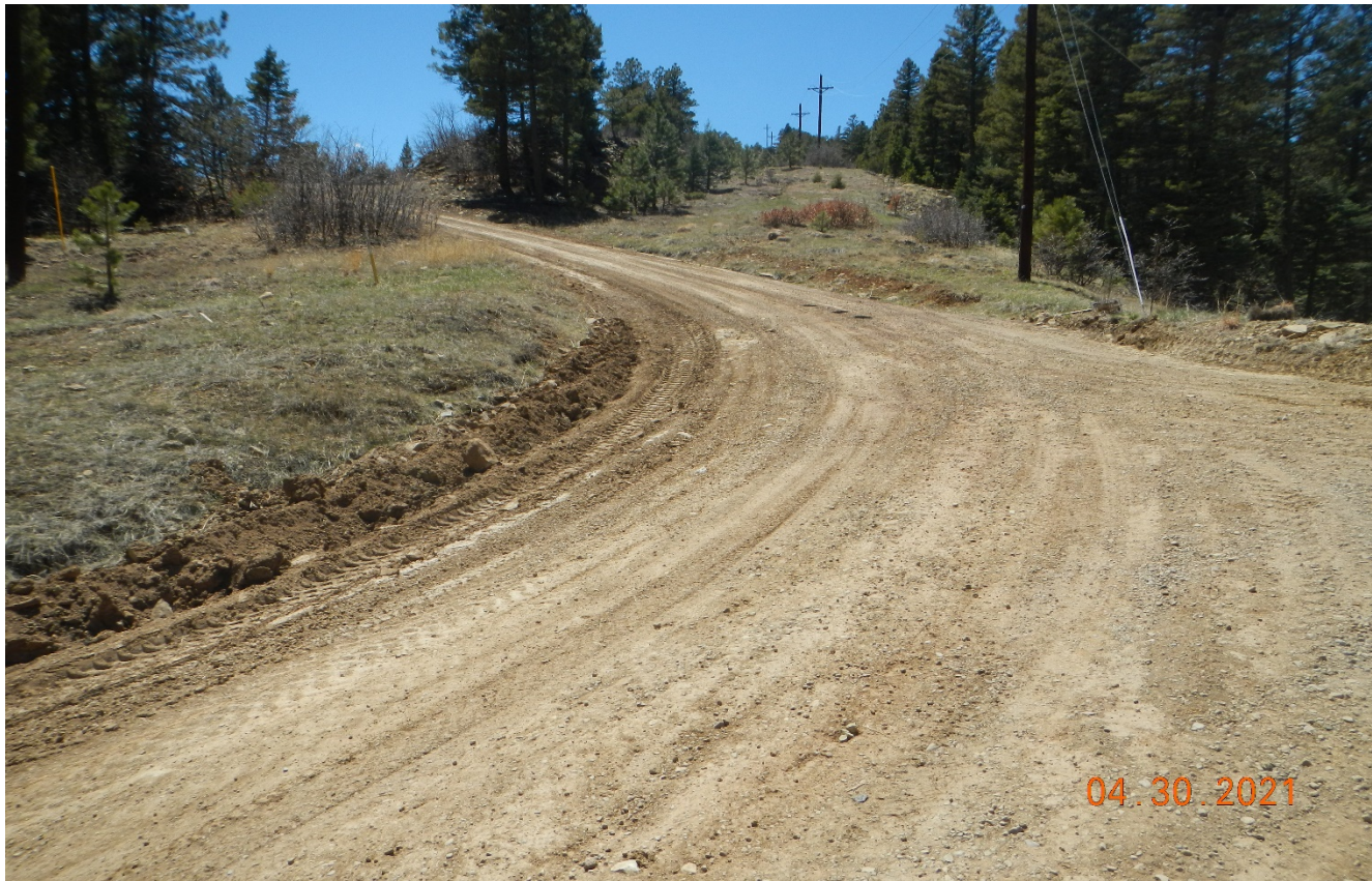
Photo 1. Facing west toward main road. The road has been regraded and repaired.
