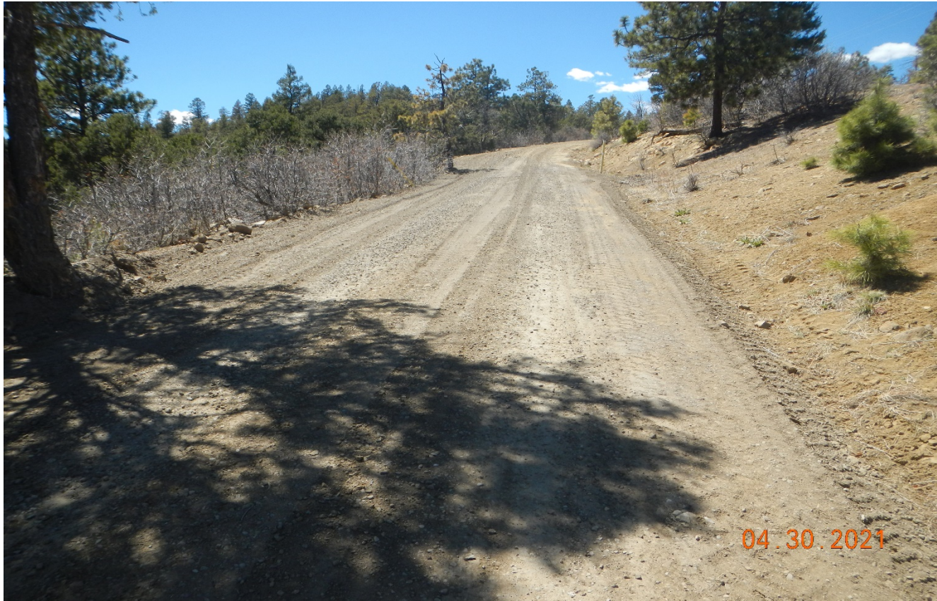
Photo 2. Areas of erosion and rutting have been repaired along the main road ascending to the hillside to the location.
