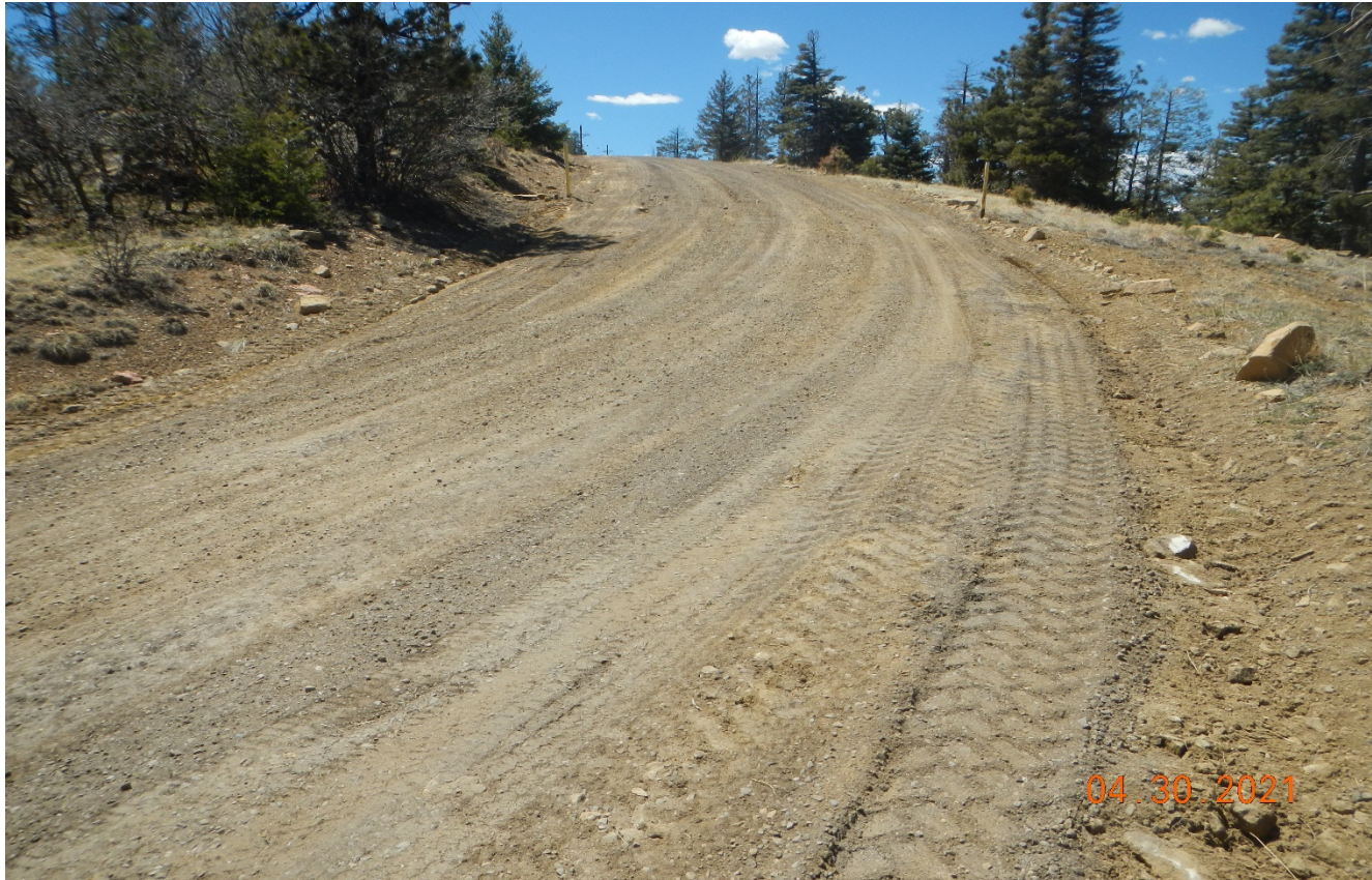
Photo 3. Areas of erosion and rutting have been repaired along the main road ascending to the hillside to the location.
