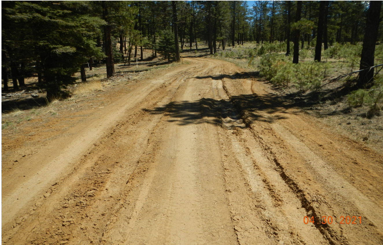
Photo 4. There is vehicle rutting along the road traveling to the location. The road needs to be maintained.
