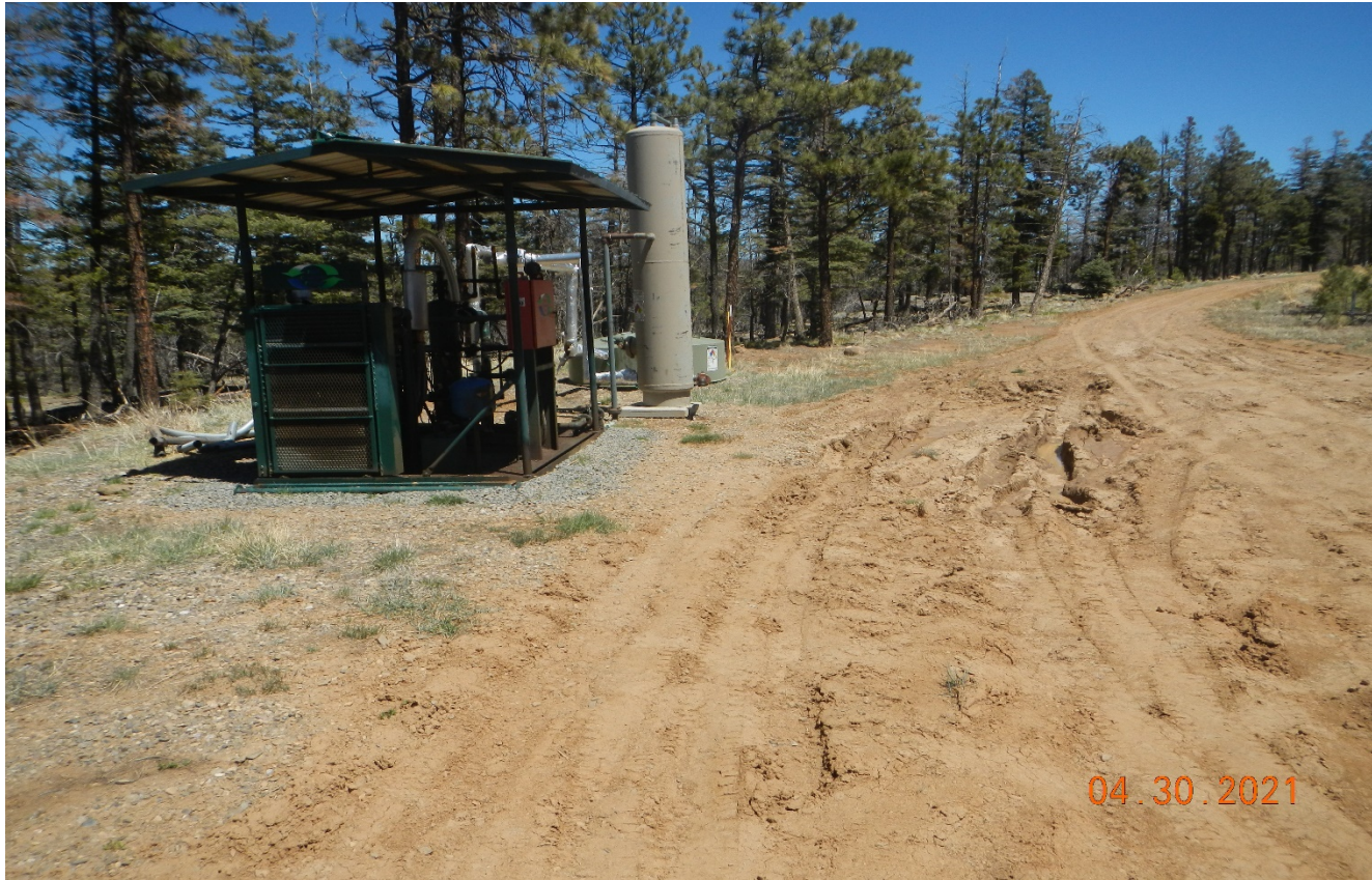
Photo 6. Facing toward the location. Areas of rutting at the location need to be repaired and stabilized.
