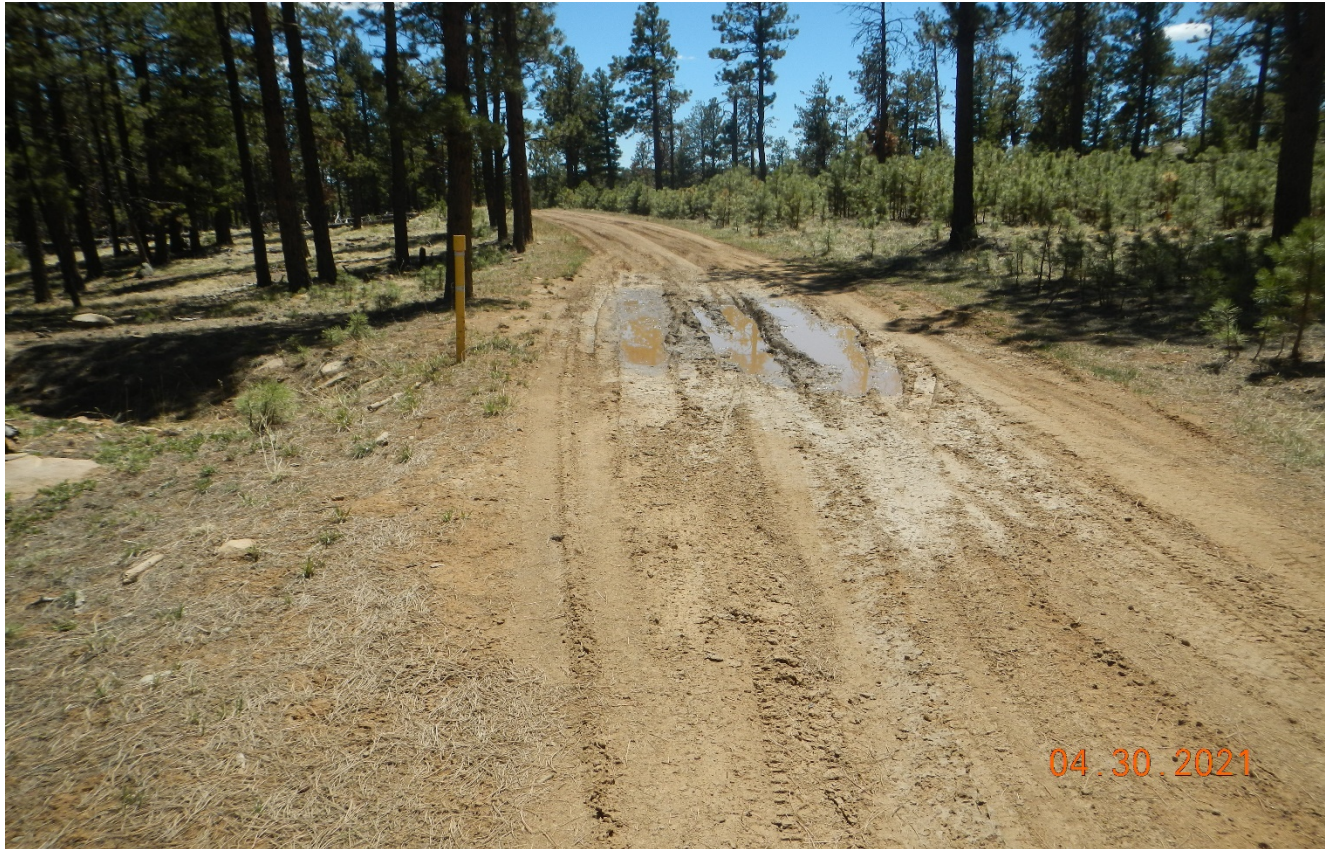
Photo 3. Likewise to previous photo. There is a low spot in the road where stormwater accumulates and vehicles are widening the road to avoid this area. This area needs to be repaired to allow proper drainage.
