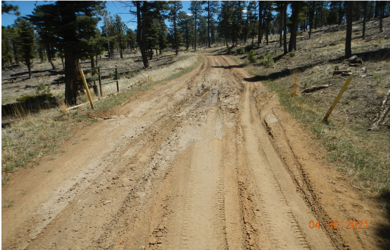
Photo 2. Facing southeast along the access road. There is a low spot in the road where stormwater accumulates. This area needs to be repaired to allow proper drainage. E.g. load of roadbase to repair and stabilize this area.
