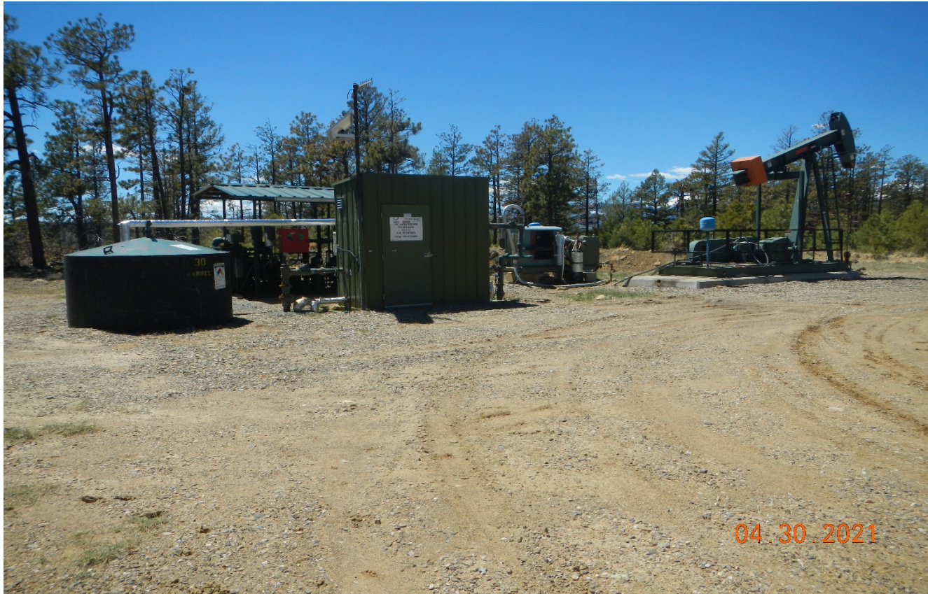
Photo 2. Well sign posted at meter shed.
