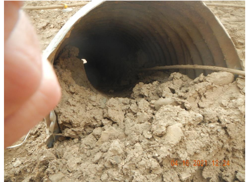
Sediment in culvert
