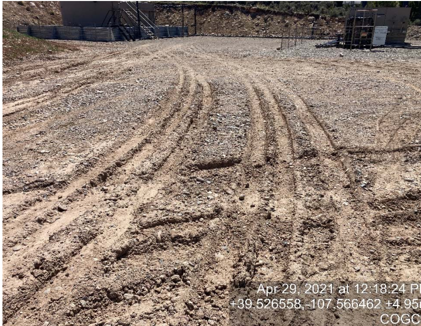
Lack of stabilization/compaction
