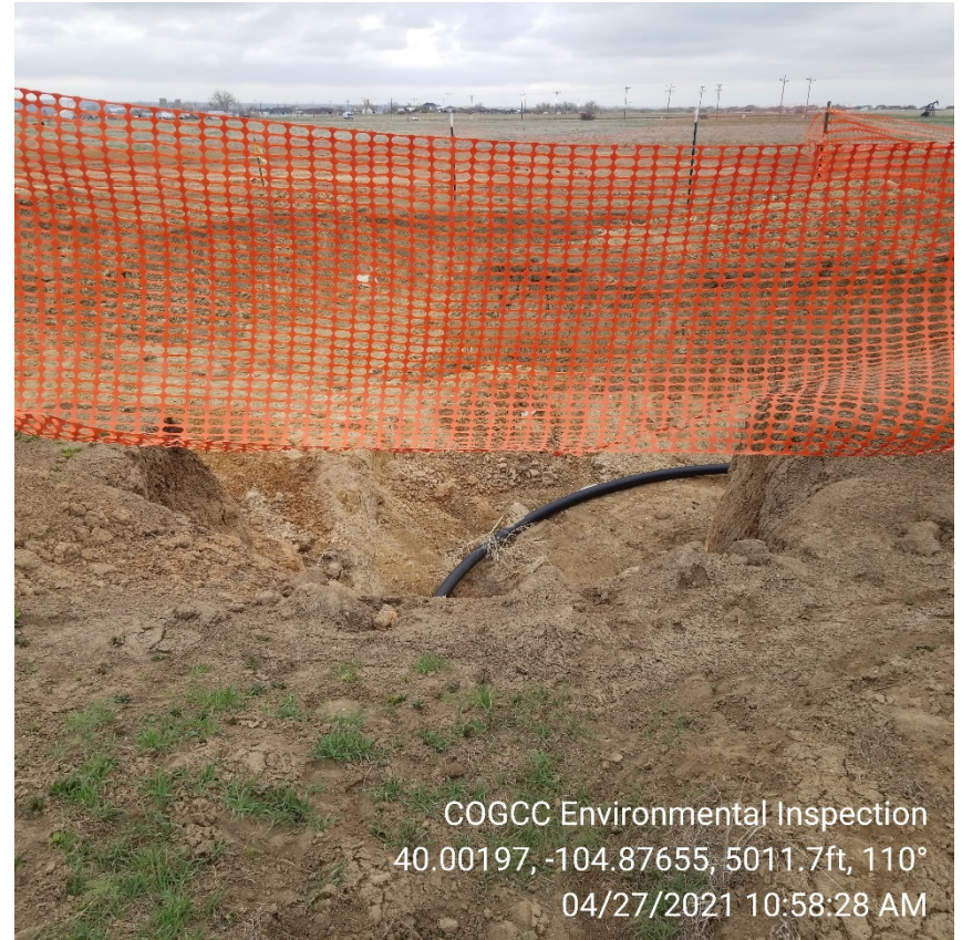
Photo 4 – Inadequate fencing with gaps
