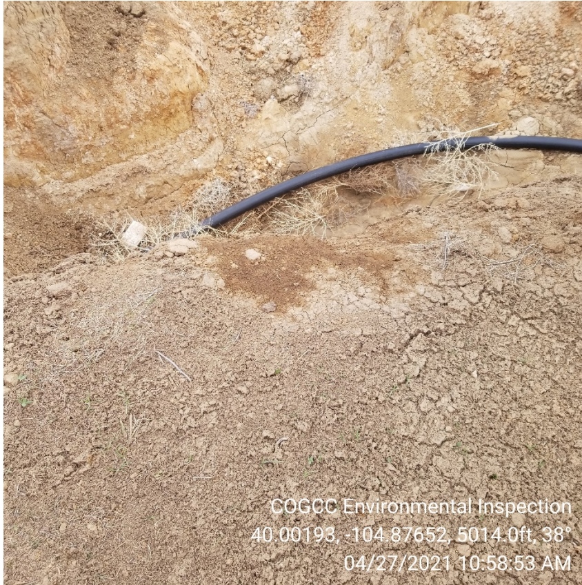
Photo 7 – Flowline and stained soil in excavation
