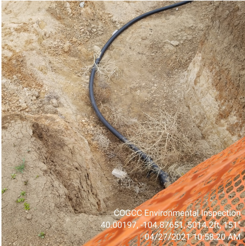
Photo 5 –Flow line visible in excavation
