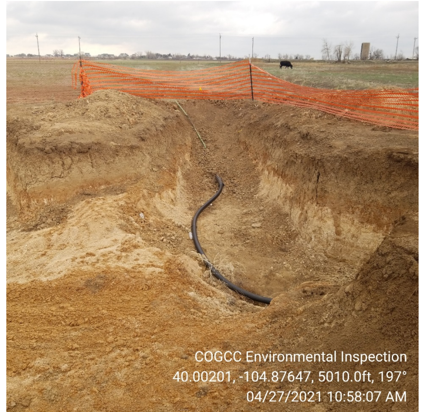
Photo 6 – Flow line visible in excavation
