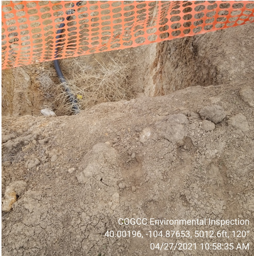
Photo 3 –Inadequate fencing with gaps
