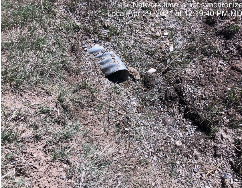
Photo #3675 Culvert capacity reduced due to inlet being crushed.
