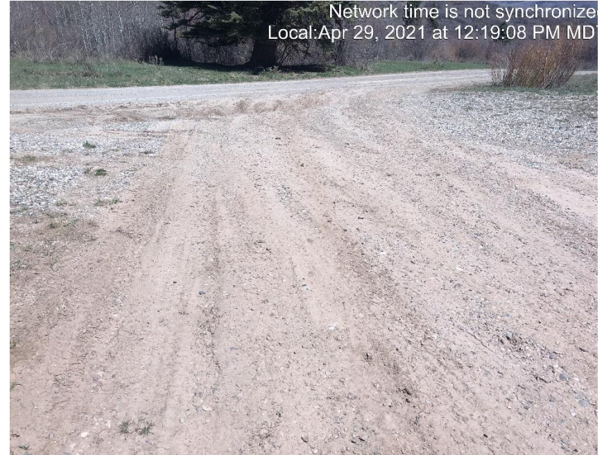
Photo #3674 No form of tracking BMP at entrance to location.
