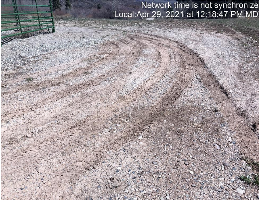
Photo #3673 location lacks stabilization.
