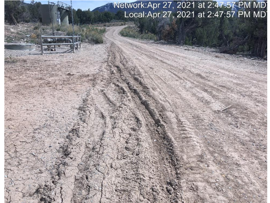
Photo #3650 No form of tracking BMP at entrance to location.
