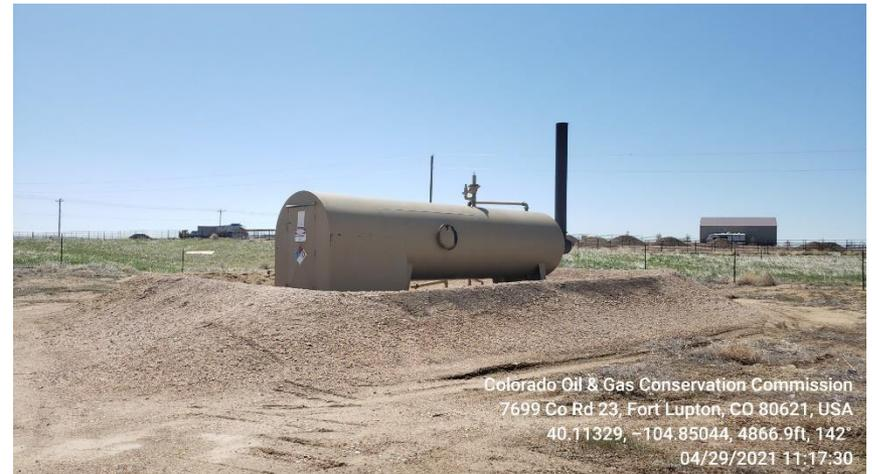
**Photo 7 Flow line manifold**
