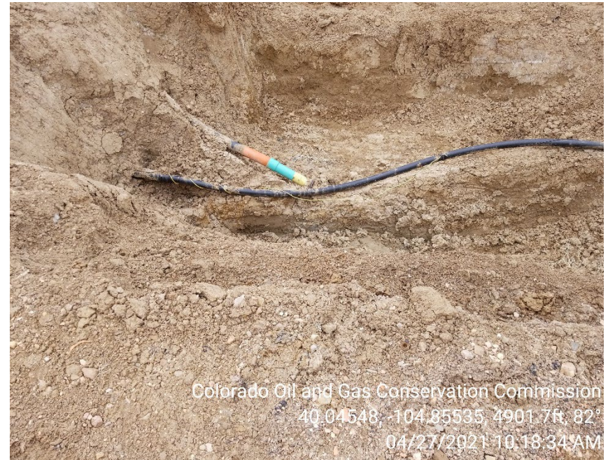
Photo 4 – Open excavation. Impacts appear to remain in situ below flowline repair.
