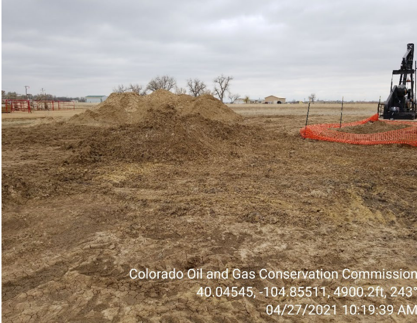
Photo 5 – Soil stored on location with inadequate BMPs.
