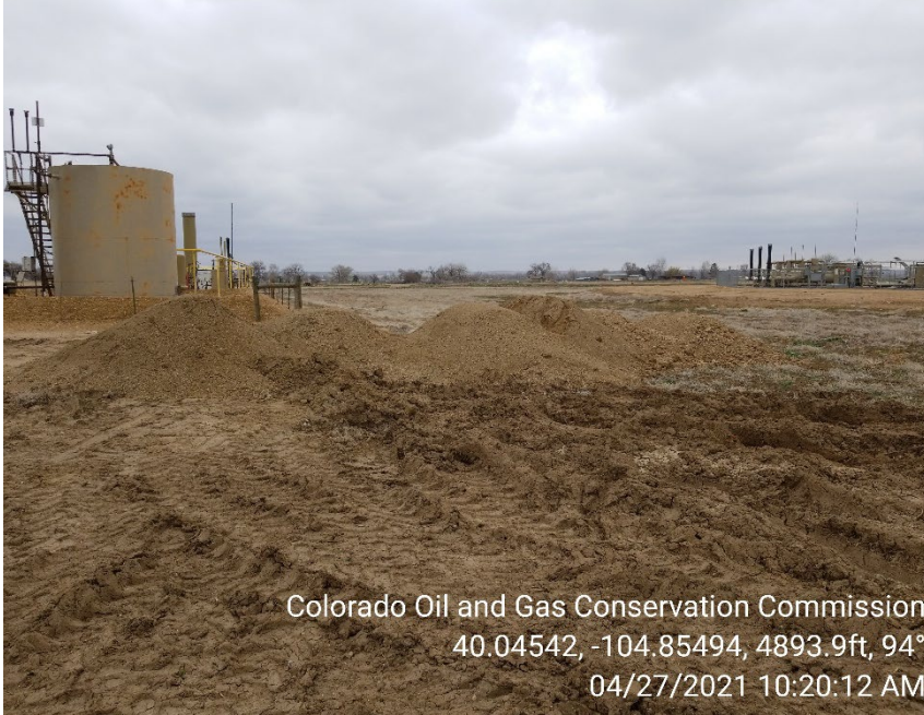
Photo 7 – Soil stored on location with inadequate BMPs.
