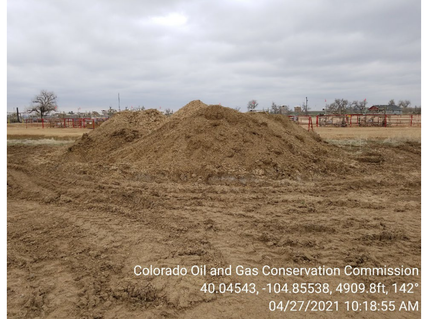
Photo 6 – Soil stored on location with inadequate BMPs.
