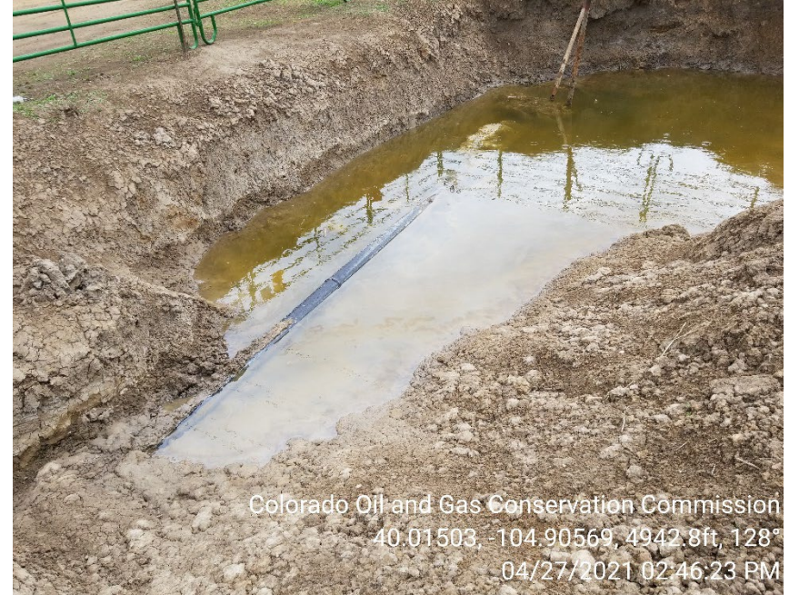
Photo 4 – Open excavation. Hydrocarbon sheen observed on groundwater.
