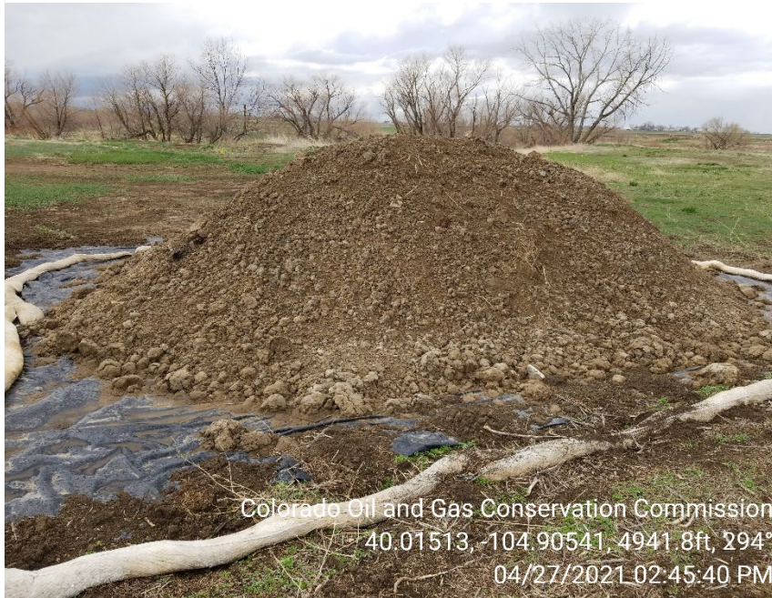
Photo 7 – BMPs are inadequate around soils stockpile.
