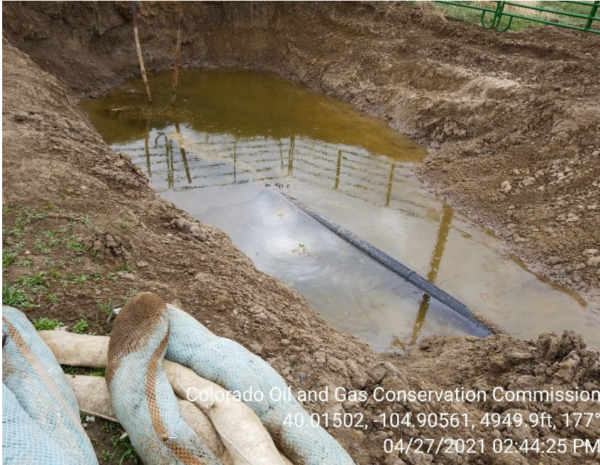
Photo 5 –Open excavation. Hydrocarbon sheen observed on groundwater.
