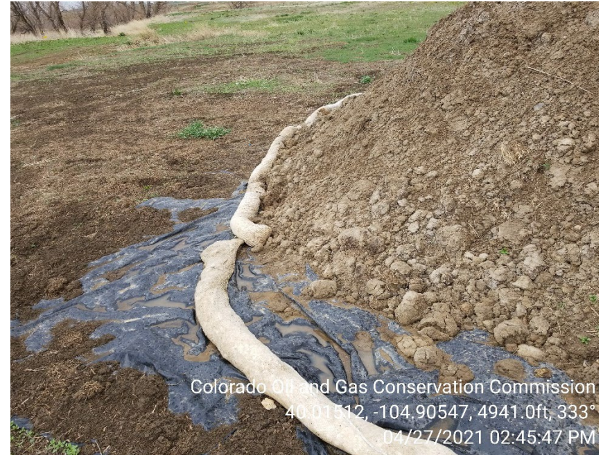
Photo 8 – BMPs are inadequate around soils stockpile.
