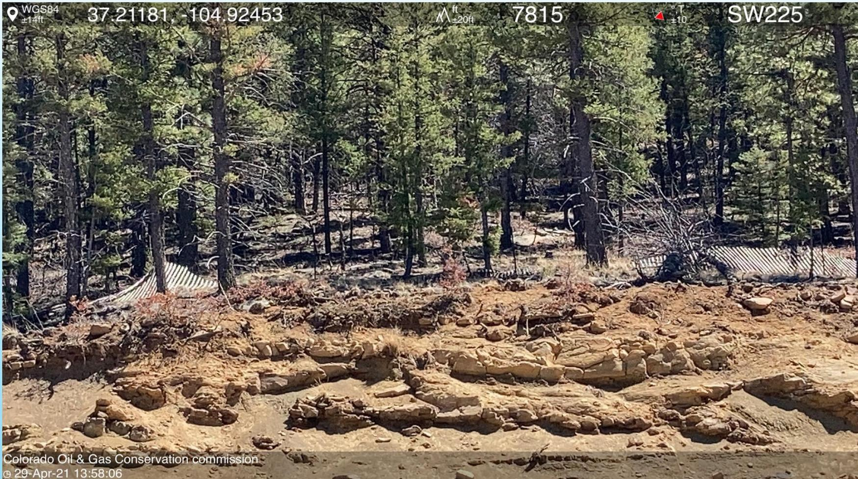
**PHOTO 4: BMP'S ARE FAILING AND IN DISREPAIR. REPAIR BMP'S. CA DATE 5-29-21.**
