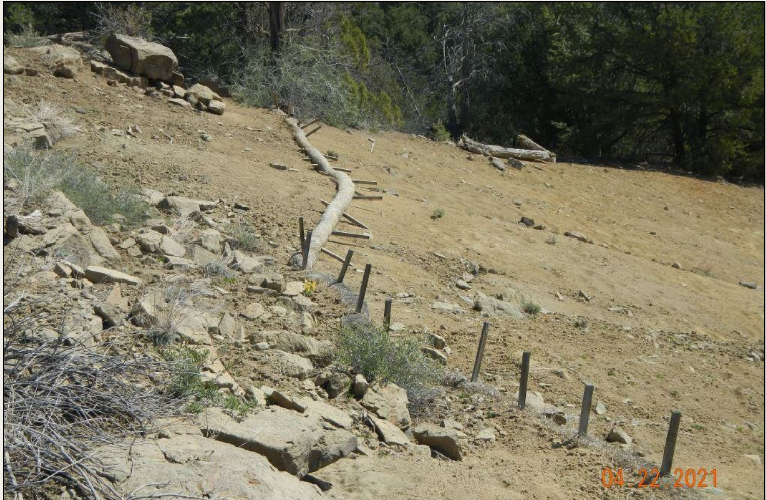
Photo 3. View of wattles at the top of the eastern cut-slope that need maintenance.
