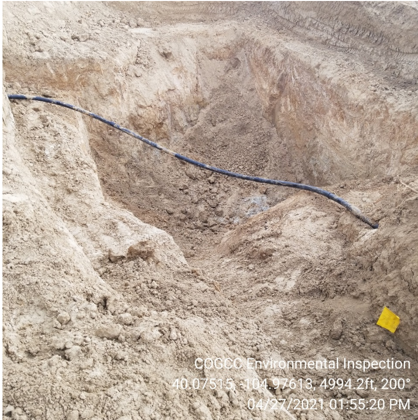
Photo 3 – Flowline visible in excavation, impacted soils visible.
