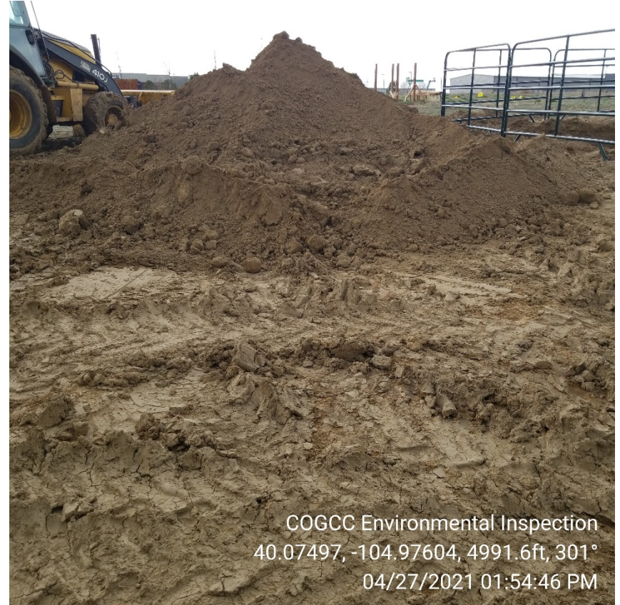
Photo 2 – Impacted soils stockpile; stormwater BMP's not correctly constructed and will channel runoff.
