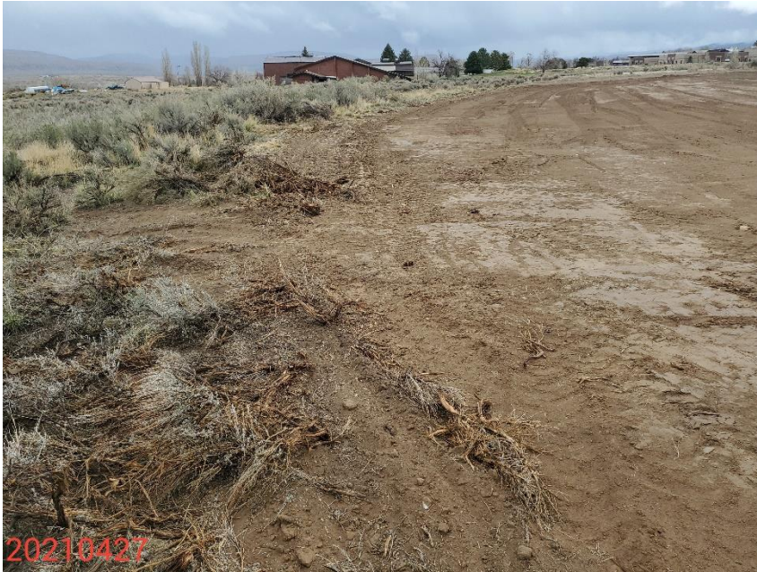
Photo 11: Photo taken from the northwestern corner of the Location, facing east. Photo shows requires stormwater and erosion control measures have not been implemented on the Location per Rules, and corrective actions.
