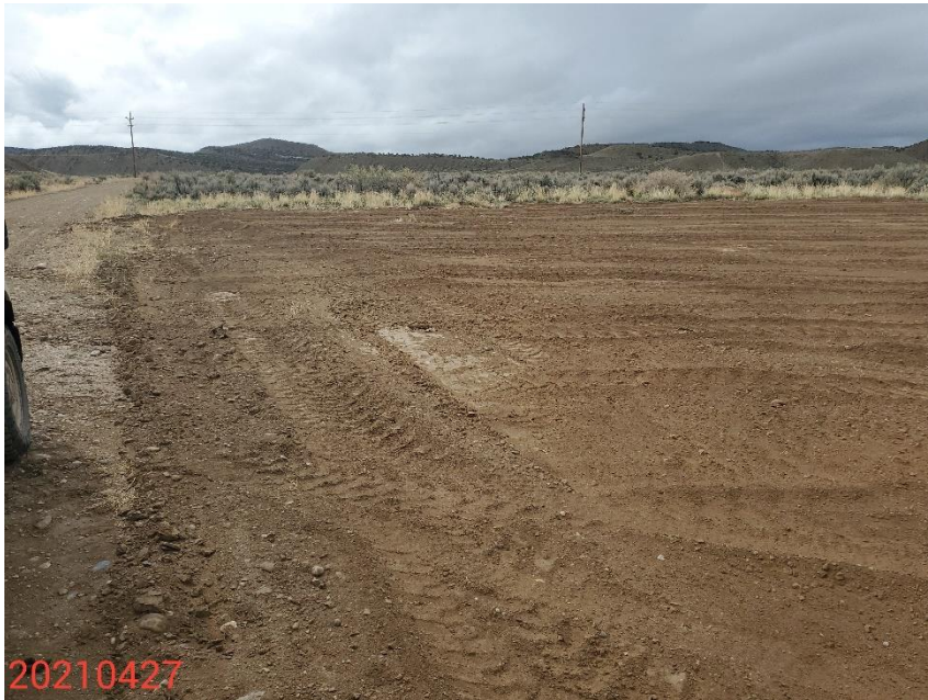
Photo 1: Photo taken from the east end of the Location, facing south. Photos 1-4 provide an overview of the Location from south, southwest, northwest to north. Photo shows additional reclamation has been performed, however, compaction issues are apparent on the Location, and stormwater control measures have not been implemented.
