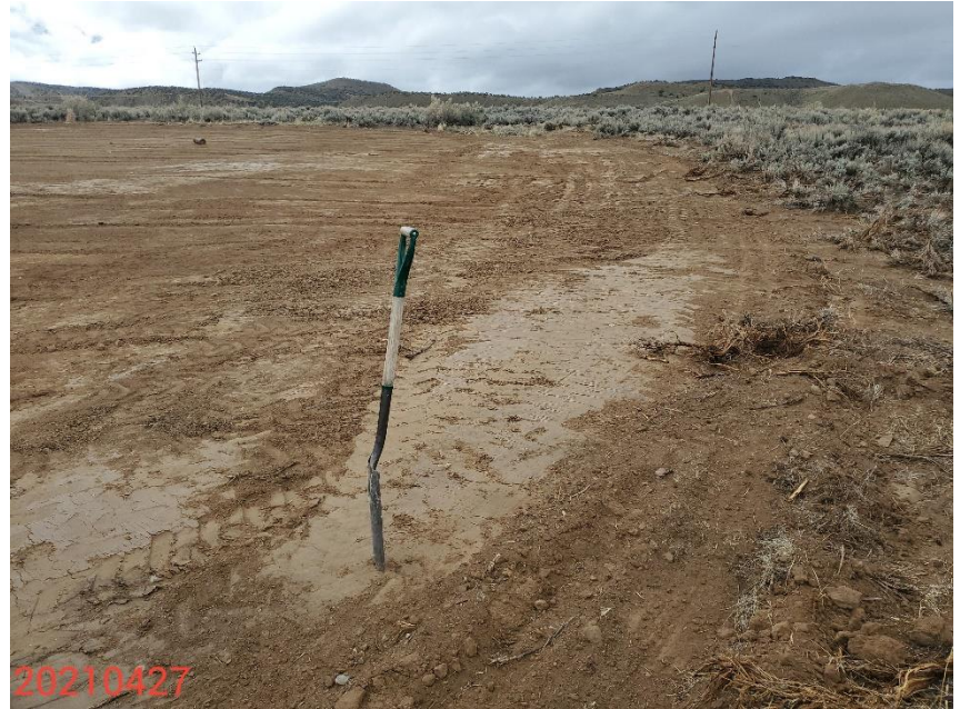
Photo 12: Photo taken from the northwestern corner of the Location, facing south. Photo shows requires stormwater and erosion control measures have not been implemented on the Location per Rules, and corrective actions.
