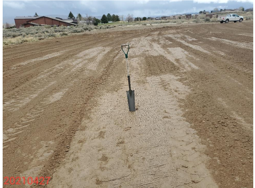
Photo 8: Photo taken from the eastern areas of the Location, facing southeast. Photo shows examples of the Location where compaction issues area apparent as the surface.
