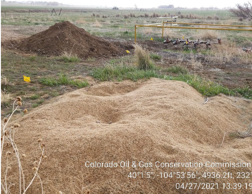
Inadequate Storm water BMPs
