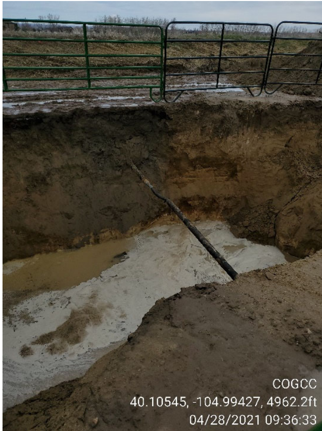
Photo 3 View of flowline repair.
