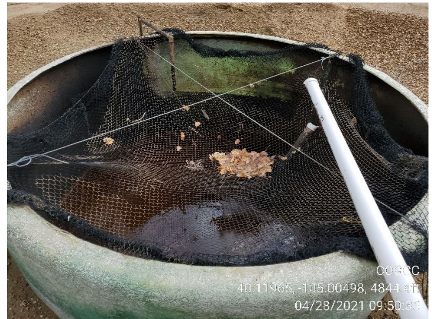
Photo 6 Partially buried produced water tank netting.
