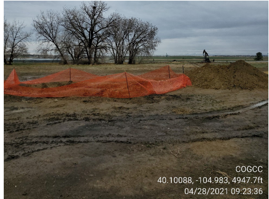
Photo 2 Excavation at flowline release point and stockpile
