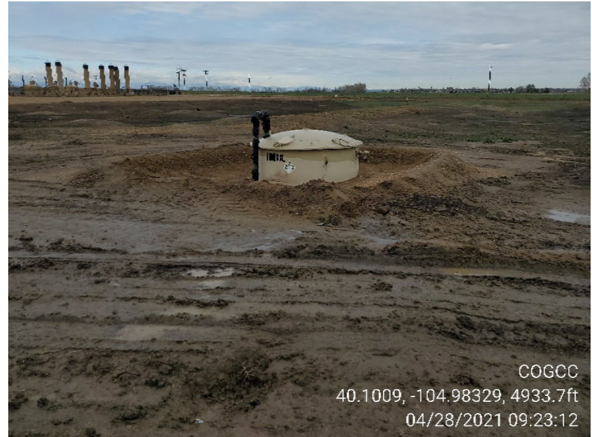
Photo 4 Partially buried vessel and secondary containment requiring maintenance
