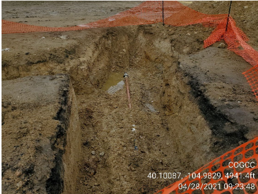
Photo 3 Exposed flowline in excavation.
