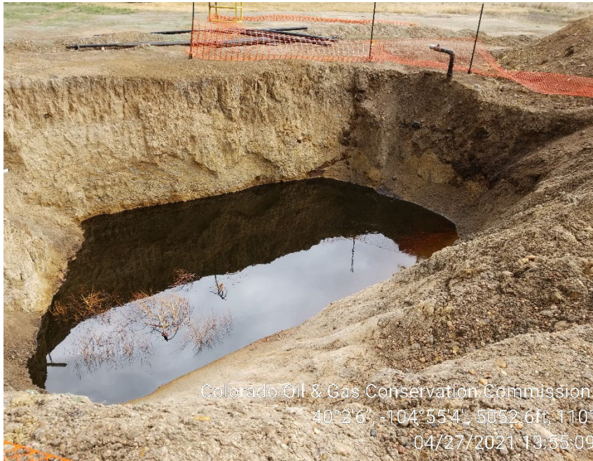
Open excavation flooded with groundwater
