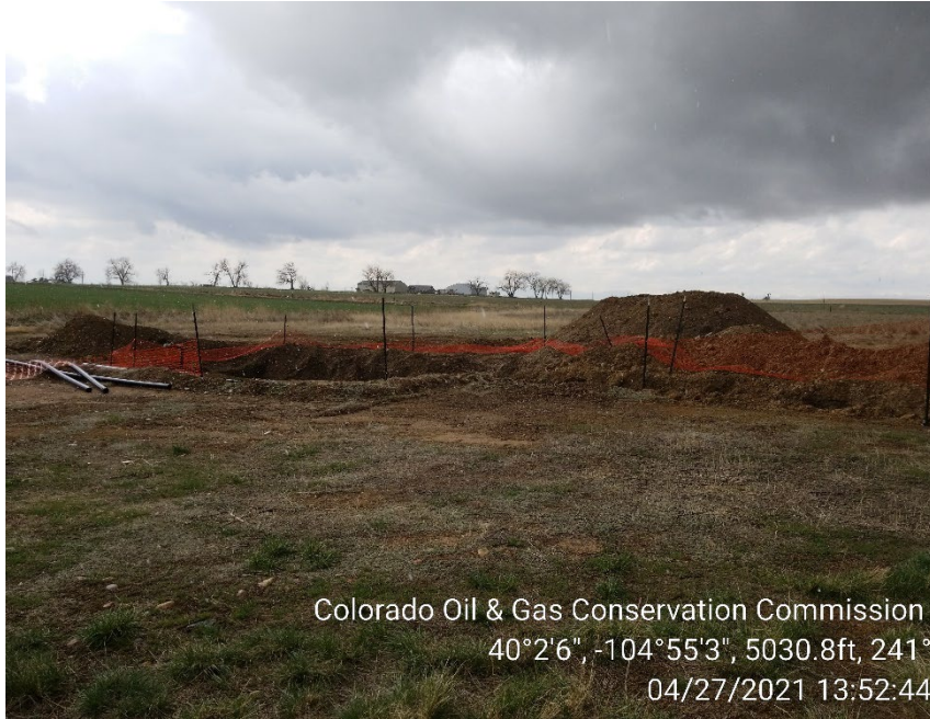
Inadequate fencing around open excavation
