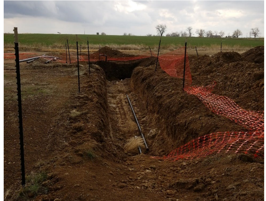
Inadequate Fencing & storm water BMPs
