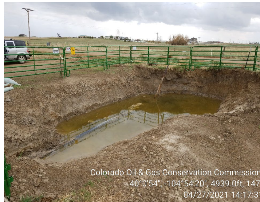
Open excavation flooded with groundwater. Gap in steel panel fencing.
