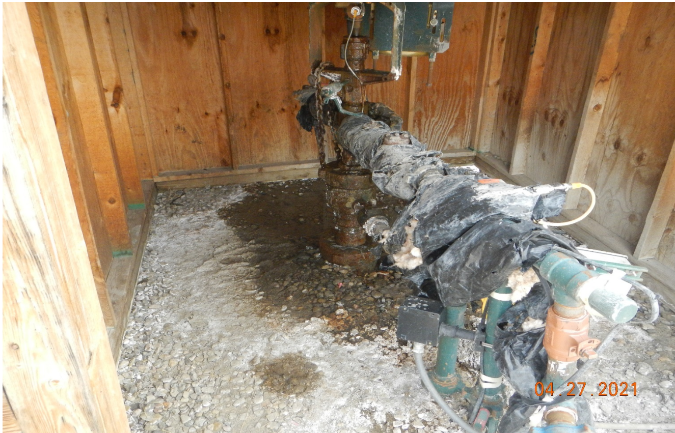
Photo 3. View of water leaking from the wellhead.
