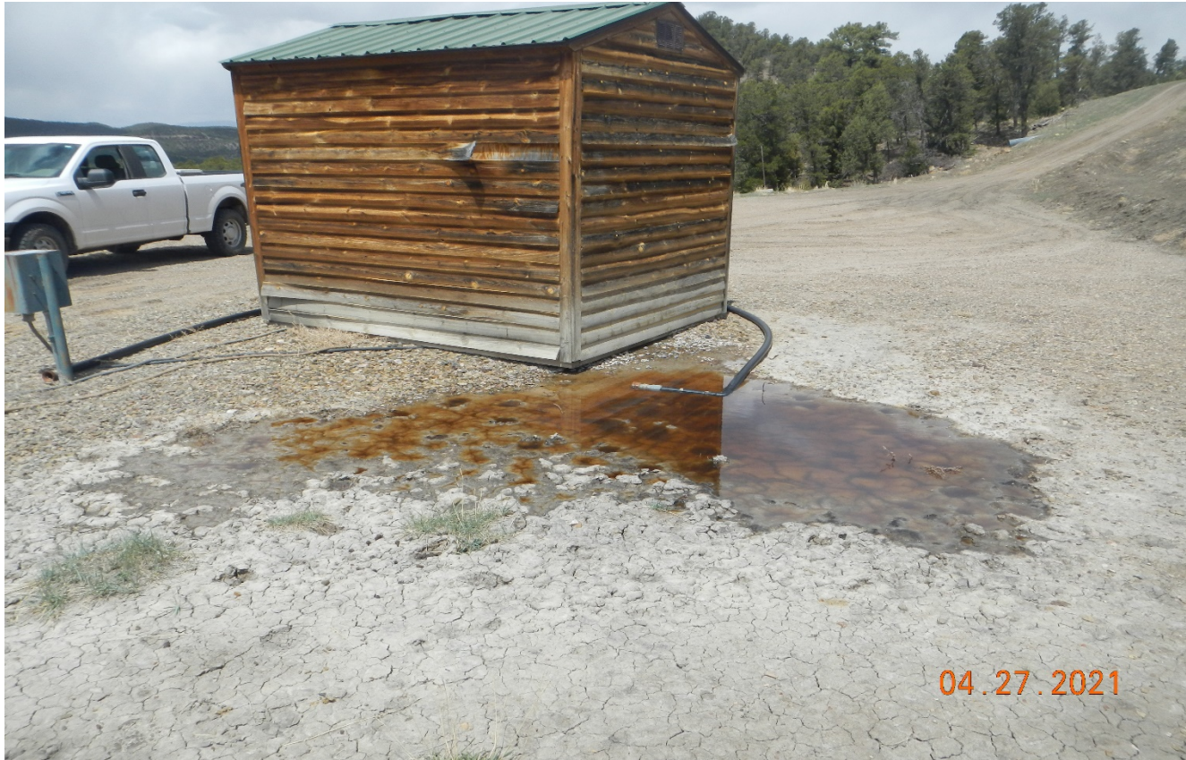
Photo 2. There is a water leak coming from the wellhead.
