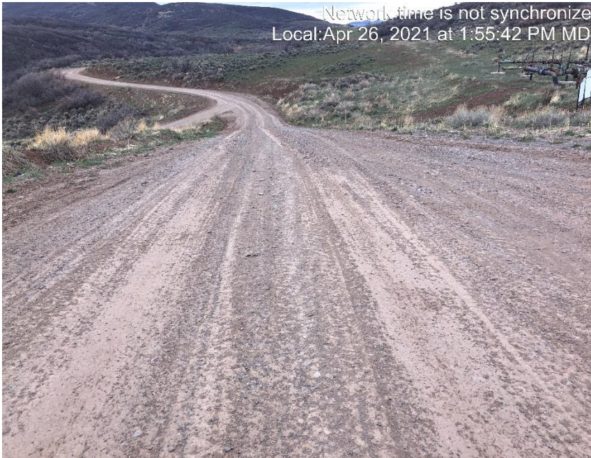
Photo #3632 No form of tracking BMP at entrance to location.
