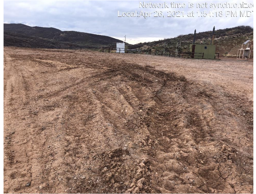
Photo #3631 Location lacks stabilization
