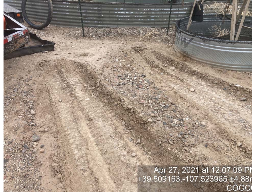
Lack of stabilization/compaction
