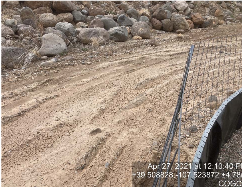
Lack of stabilization/compaction
