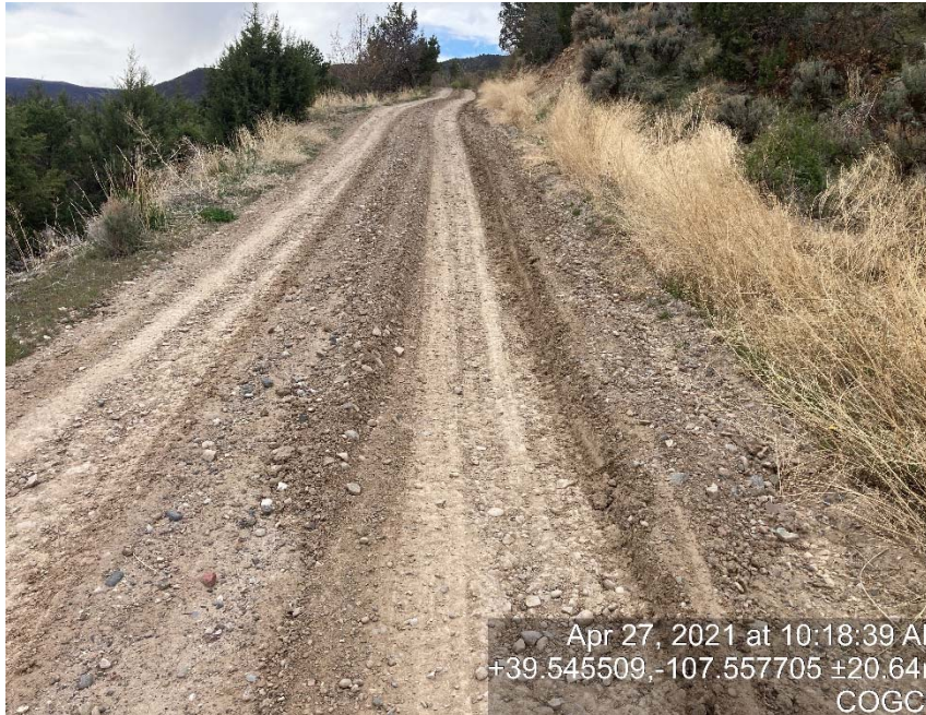
Lack of stabilization/compaction on access road
