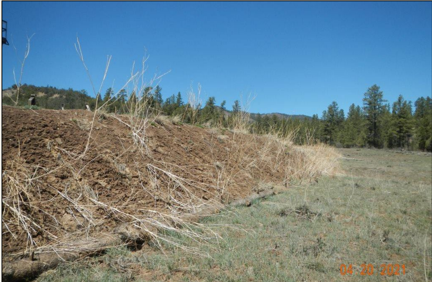
Photo 2. View of the eastern fill slope from the southeastern corner facing northward. Revegetation is in an early reclamation condition. Small grasses such as squirreltail and western wheatgrass, as well as clover (likely melilotus) observed within the reclamation areas.
