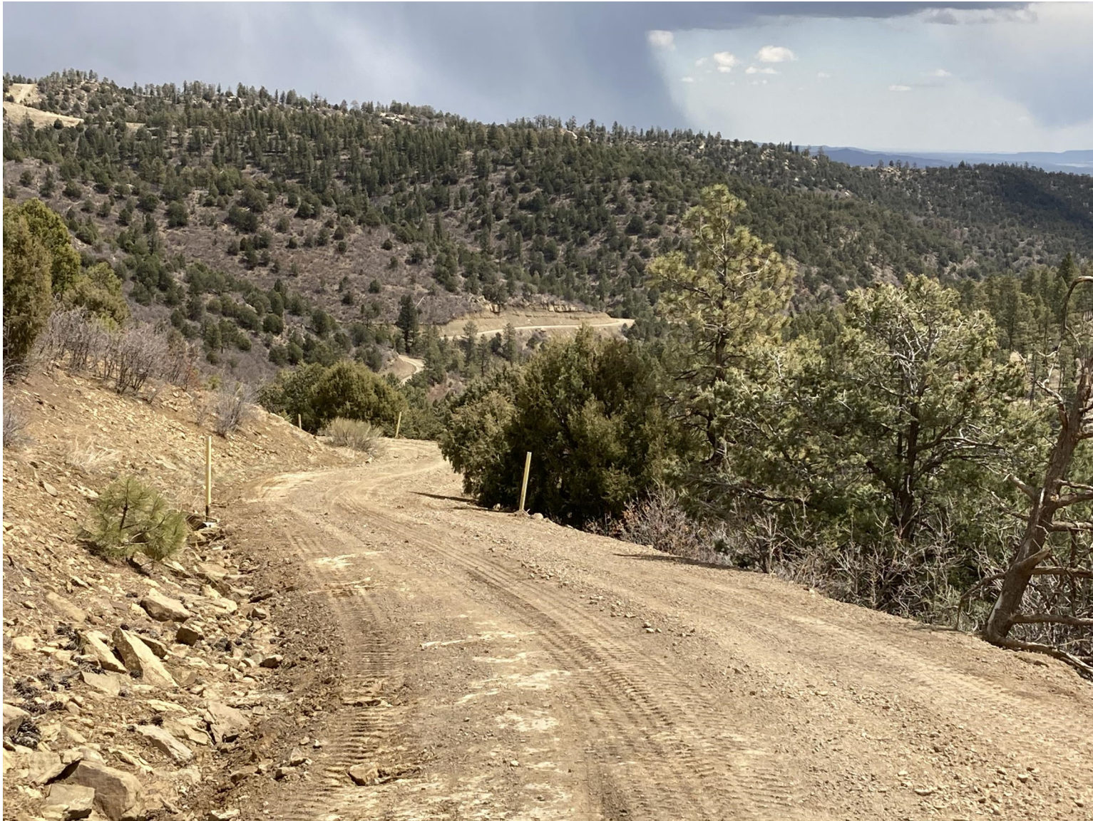
PHOTO 11: THE MAIN LEASE ROAD SURFACE WAS CROWNED TO REMOVE THE SURFACE EROSION.
