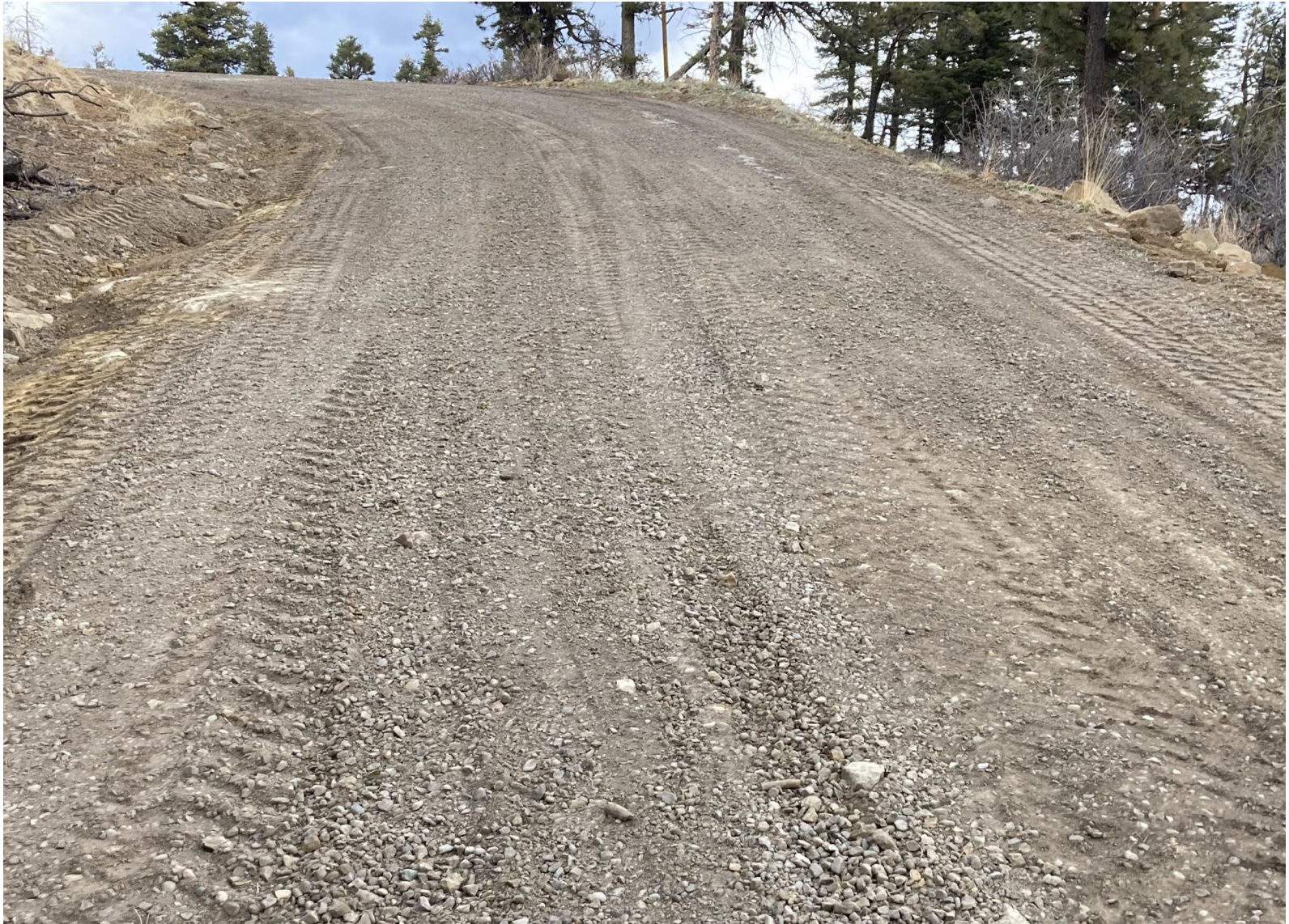
PHOTO 8: THE MAIN LEASE ROAD SURFACE WAS CROWNED TO REMOVE THE SURFACE EROSION.
