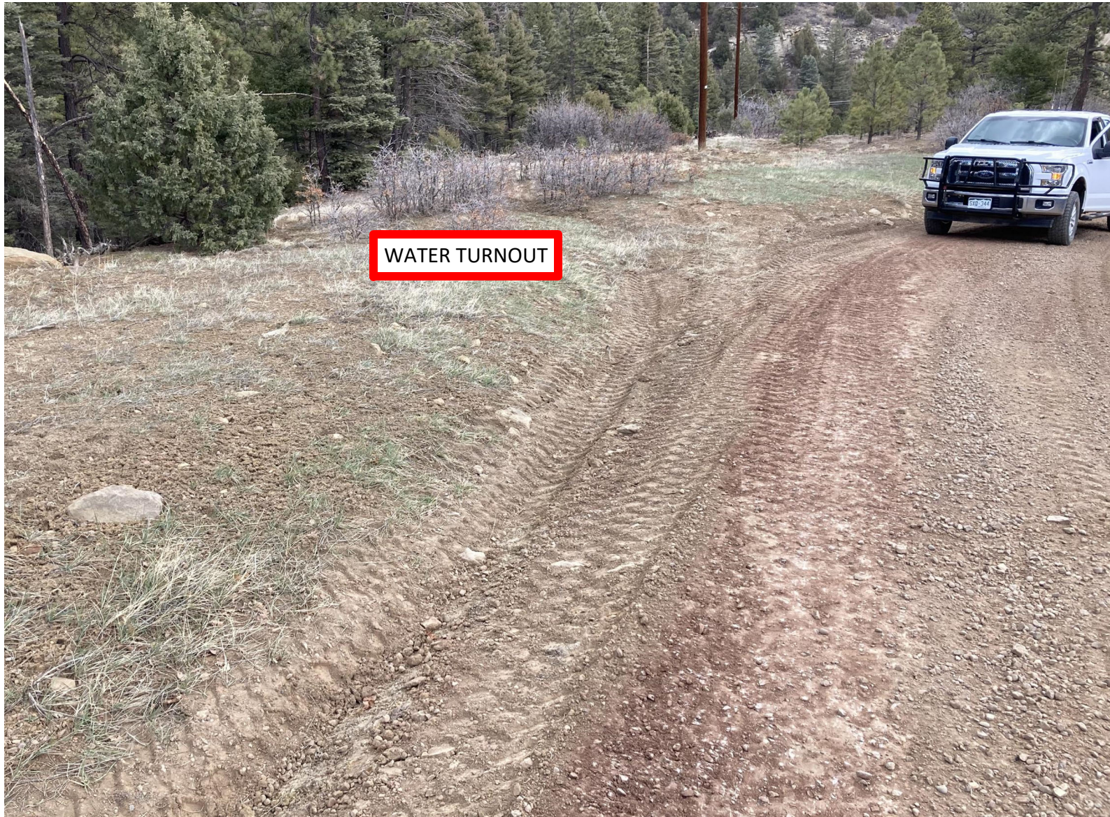
PHOTO 5: THE MAIN LEASE ROAD SURFACE WAS CROWNED TO REMOVE THE TIRE RUTS AND ESTABLISH SHEET FLOW. WATER TURNOUTS WERE INSTALLED TO REMOVE WATER FROM THE BAR DITCH REDUCING THE VOLUME AND THE VELOCITY OF THE RUN OFF.
