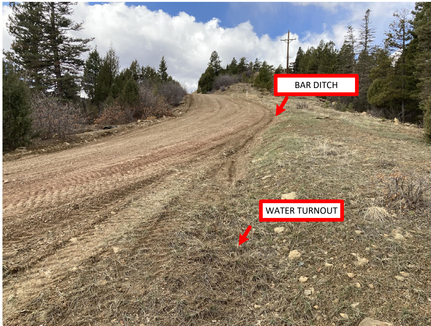
PHOTO 4: THE MAIN LEASE ROAD SURFACE WAS CROWNED TO REMOVE THE TIRE RUTS AND ESTABLISH SHEET FLOW. WATER TURNOUTS WERE INSTALLED TO REMOVE WATER FROM THE BAR DITCH REDUCING THE VOLUME AND THE VELOCITY OF THE RUN OFF.
