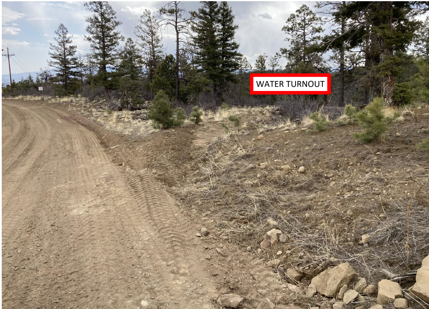
PHOTO 9: THE MAIN LEASE ROAD SURFACE WAS CROWNED TO REMOVE THE TIRE RUTS AND ESTABLISH SHEET FLOW. WATER TURNOUTS WERE INSTALLED TO REMOVE WATER FROM THE BAR DITCH REDUCING THE VOLUME AND THE VELOCITY OF THE RUN OFF.
