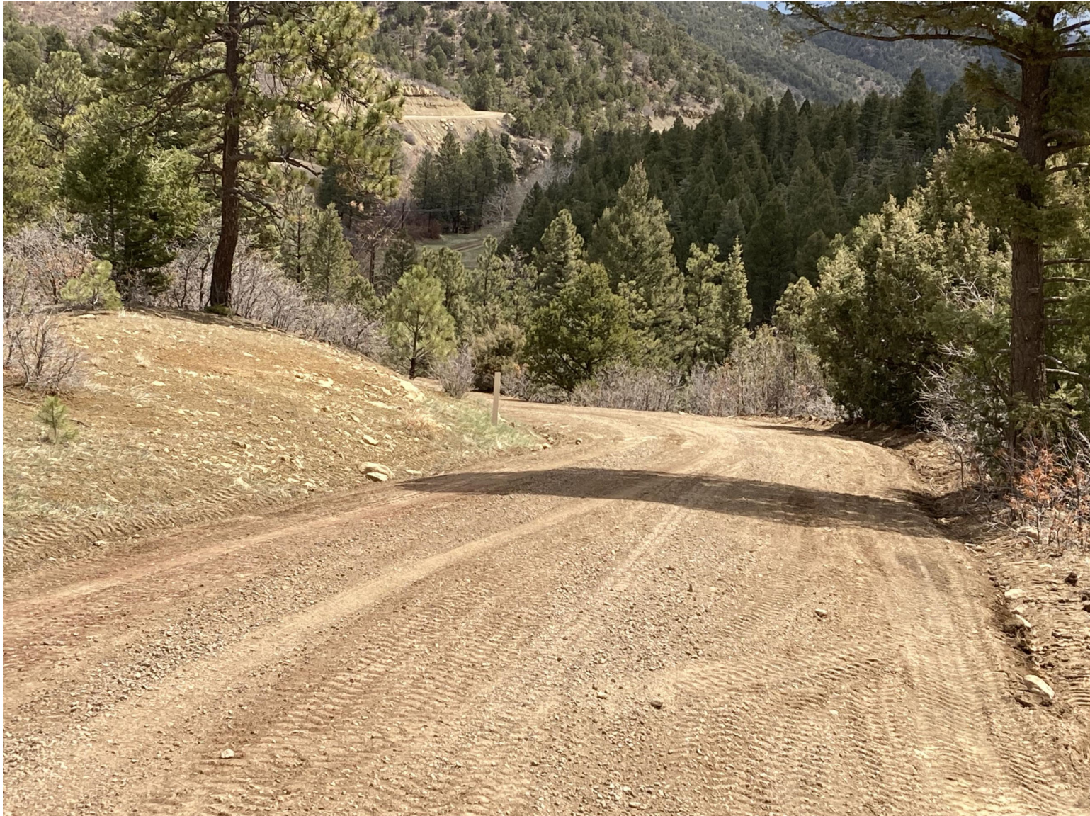
PHOTO 12: THE MAIN LEASE ROAD SURFACE WAS CROWNED TO REMOVE THE SURFACE EROSION.
