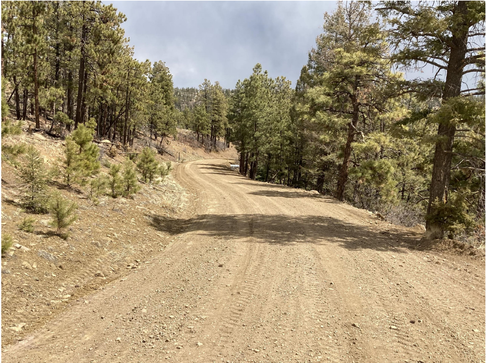
PHOTO 10: THE MAIN LEASE ROAD SURFACE WAS CROWNED TO REMOVE THE SURFACE EROSION.
