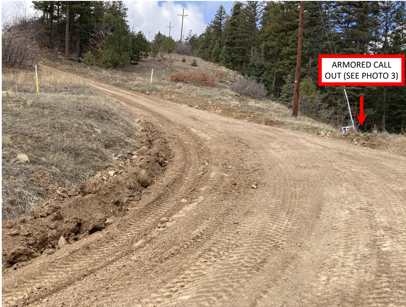
PHOTO 2: THE MAIN LEASE ROAD SURFACE WAS CROWNED TO REMOVE THE SURFACE EROSION AND ESTABLISH SHEET FLOW. THE BAR DITCH WAS DOMINATED TO RECEIVE STORMWATER ON THE NORTH SIDE OF THE ROAD TO DIRECT RUN OFF TO AN ARMORED CALL OUT, WHICH DRAINS INTO AN EXISTING SEDIMENT BASIN.
