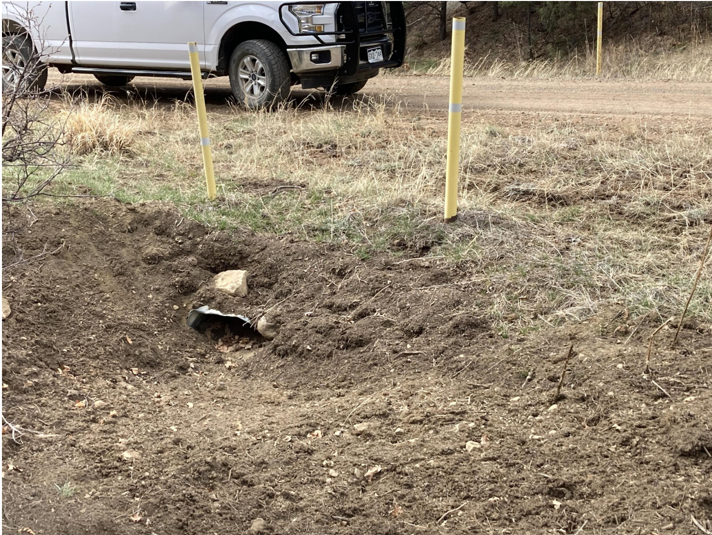
PHOTO 1: THE SEDIMENT ACCUMULATION WAS REMOVED FROM THE CULVERT INLET.
