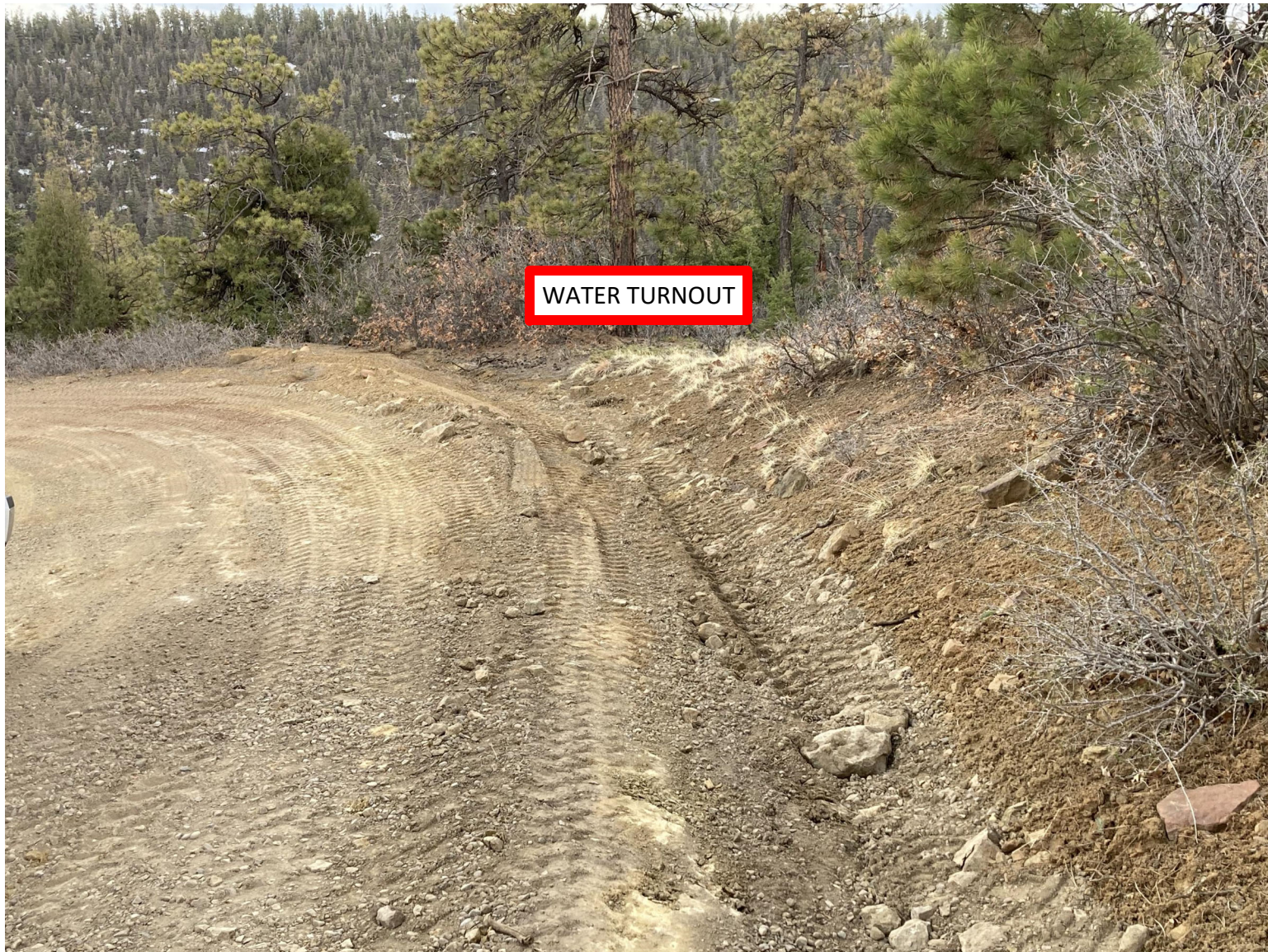
PHOTO 7: THE MAIN LEASE ROAD SURFACE WAS CROWNED TO REMOVE THE TIRE RUTS AND ESTABLISH SHEET FLOW. WATER TURNOUTS WERE INSTALLED TO REMOVE WATER FROM THE BAR DITCH REDUCING THE VOLUME AND THE VELOCITY OF THE RUN OFF.
