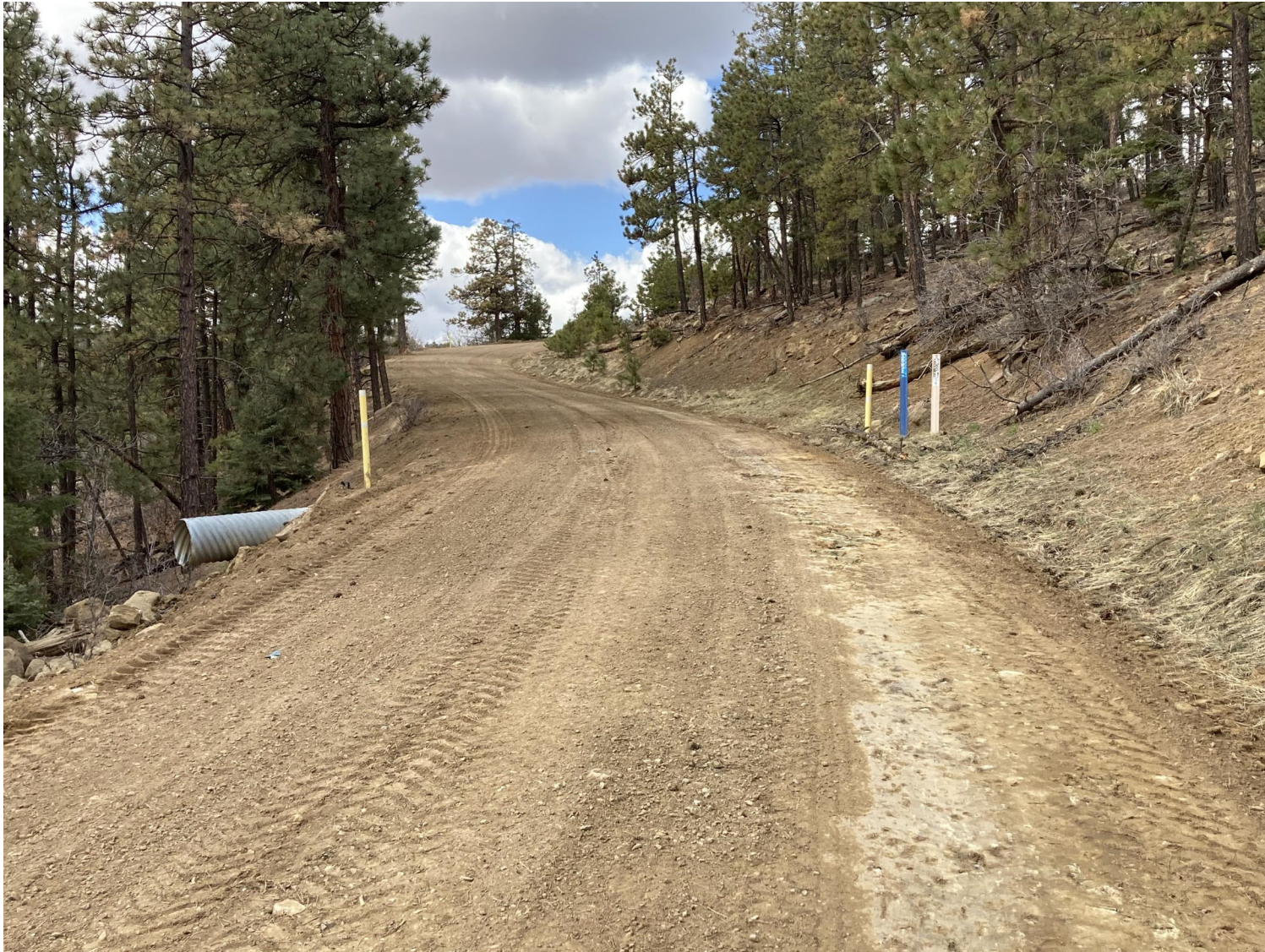
PHOTO 6: THE MAIN LEASE ROAD SURFACE WAS CROWNED TO REMOVE THE SURFACE EROSION.
