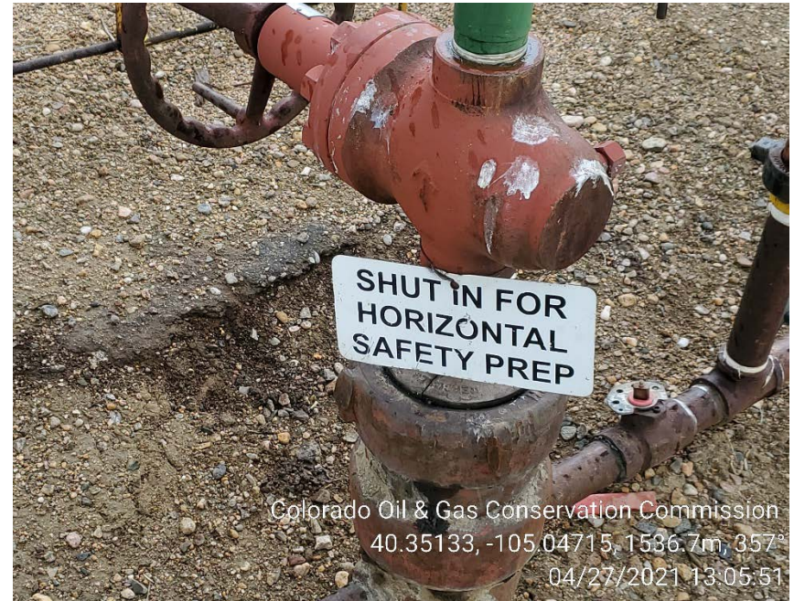
HZ safety prep sign
