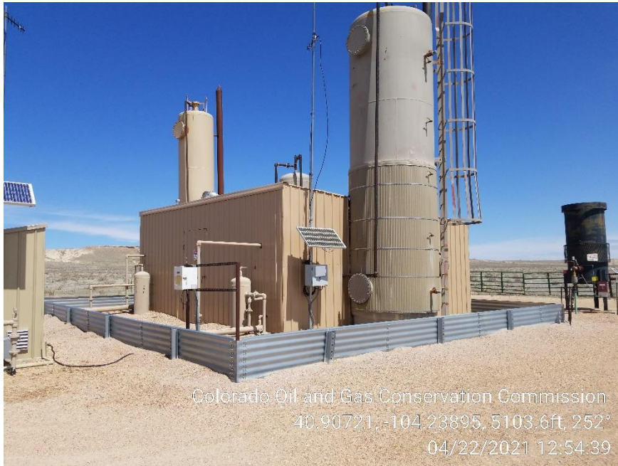
Photo 1 – Heater Treater and ECD
