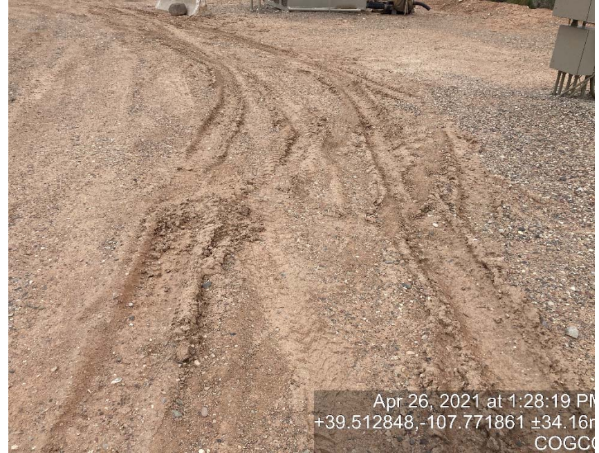
Lack of stabilization/compaction
