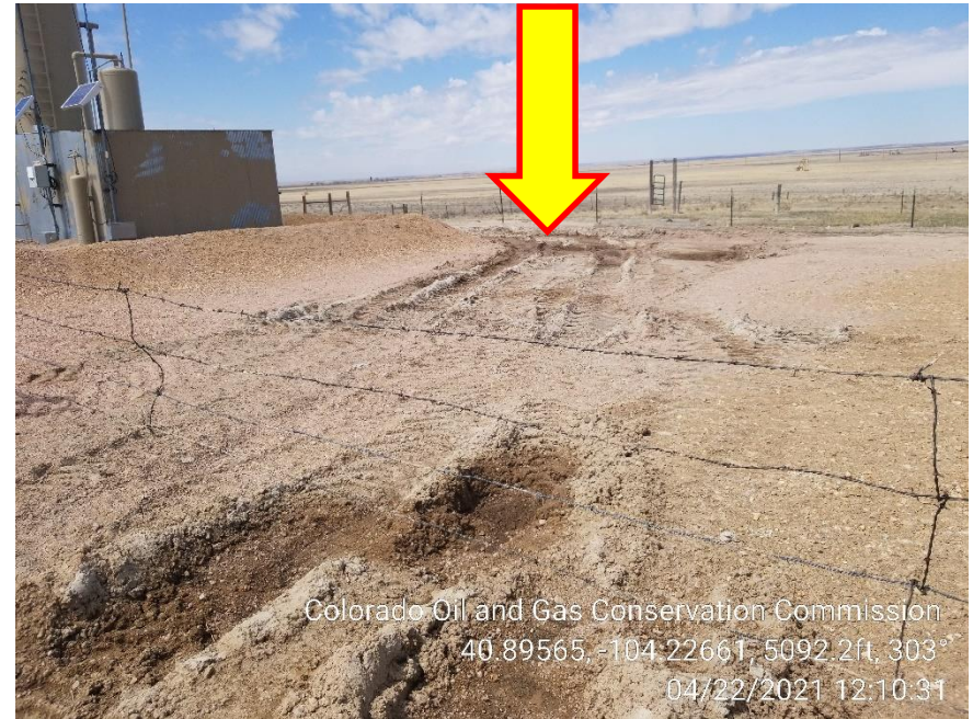
Photo 6 – Storm Water erosion
