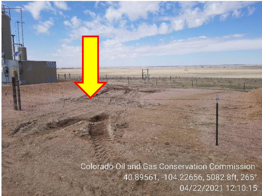
Photo 5 – Storm Water erosion
