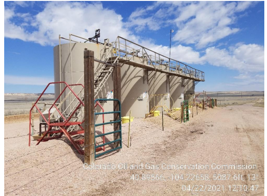
Photo 2 – Tank Battery
