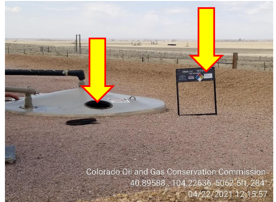
Photo 4 – Capacity Label Fading and Lid needs replaced
