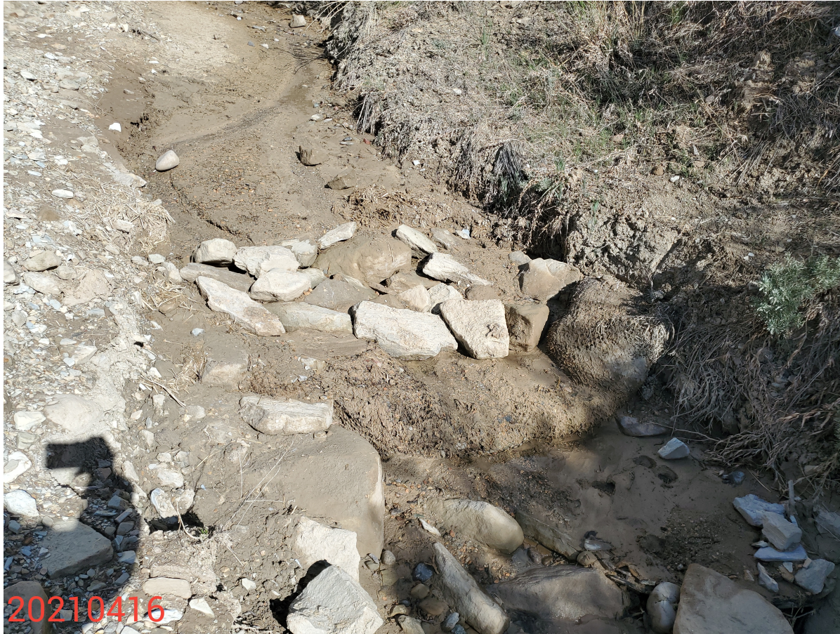
Photo 32: Photo taken downstream from the road crossing. Photo shows wattle control measure within channel that has filled with sediment and requires removal.
