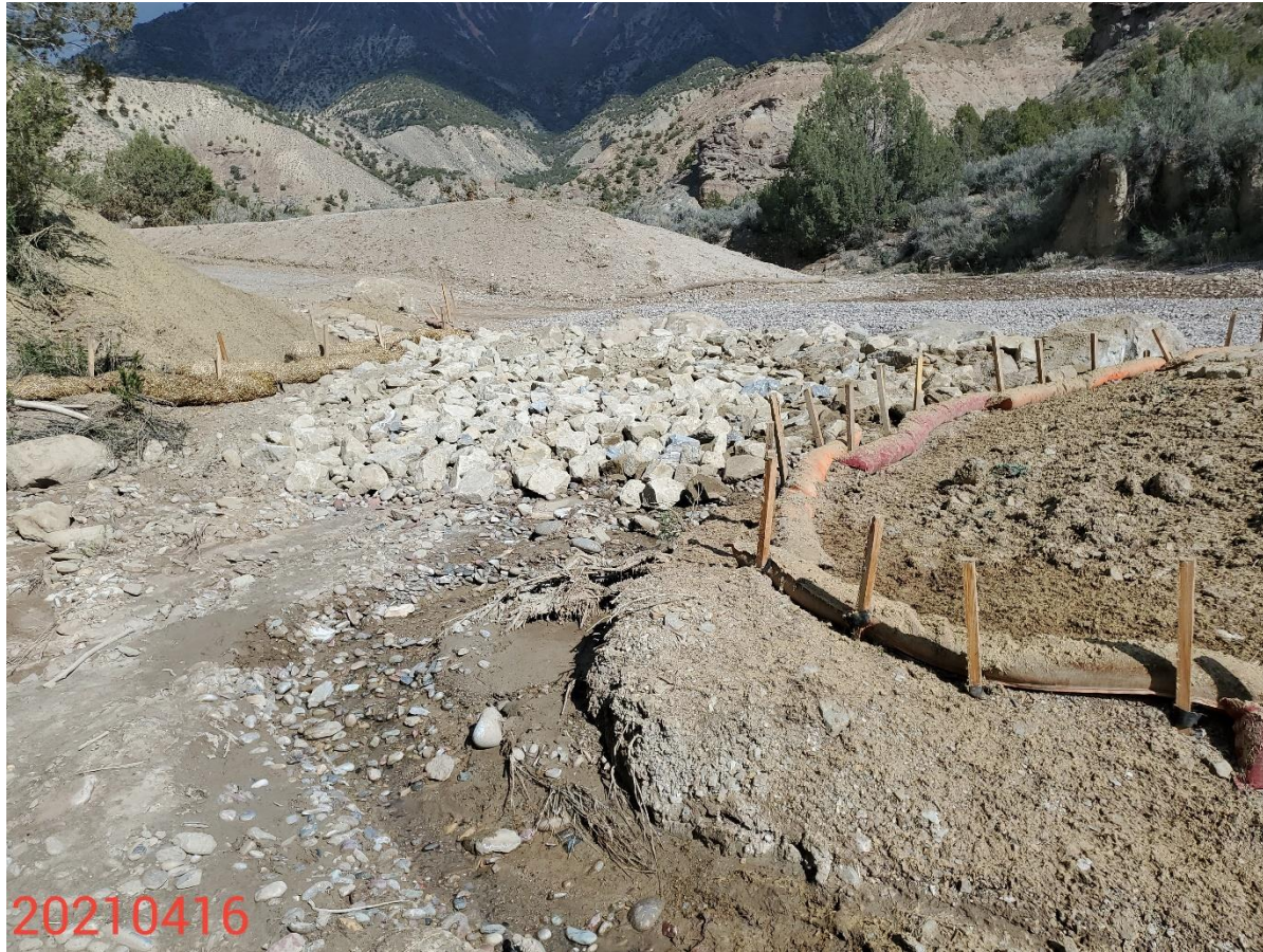
Photo 31: Photo taken downstream from the road crossing, facing north (upstream).
