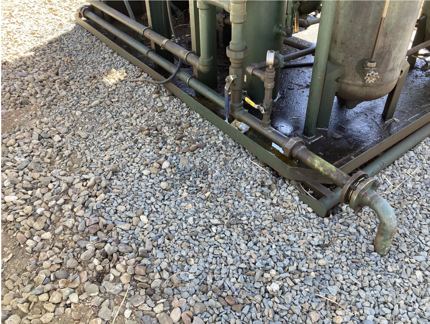
PHOTO 6: THE FLUID ACCUMULATION THAT WAS FOUND INSIDE OF THE CONTAINMENT SKID OF THE LIQUID RING COMPRESSOR WAS REMOVED.
