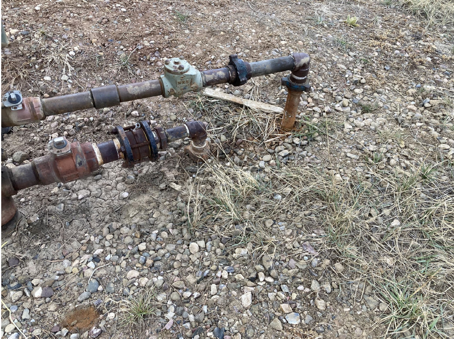
PHOTO 3: THE DISCONNECTED WATER LINE FROM THE WELL HEAD WAS RECONNECTED AND THE POLY PIPE TO THE PIT WAS REMOVED.
