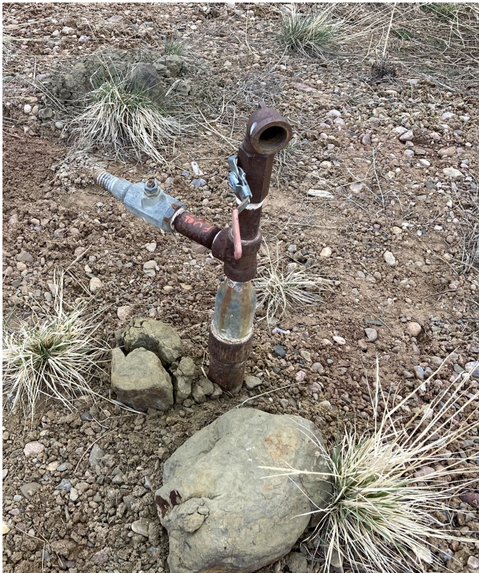
PHOTO 2: THE RISER WAS LABELED AS THE FUEL GAS LINE.
