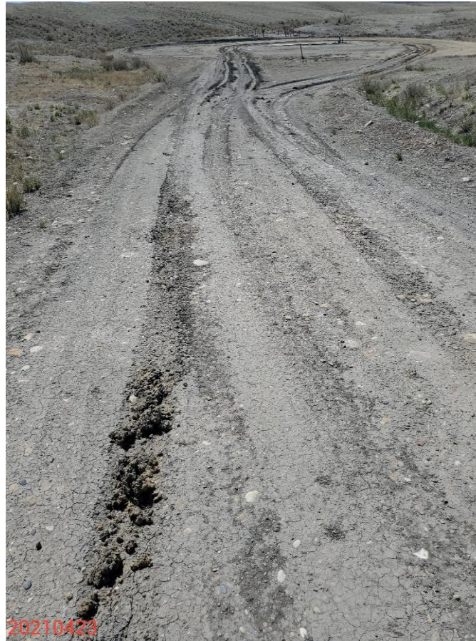
Photo 8: Photo taken from the access, facing south. Photo shows control measures to stabilize the production areas, and prevent off-site sediment transport during wet conditions are missing or insufficient.
