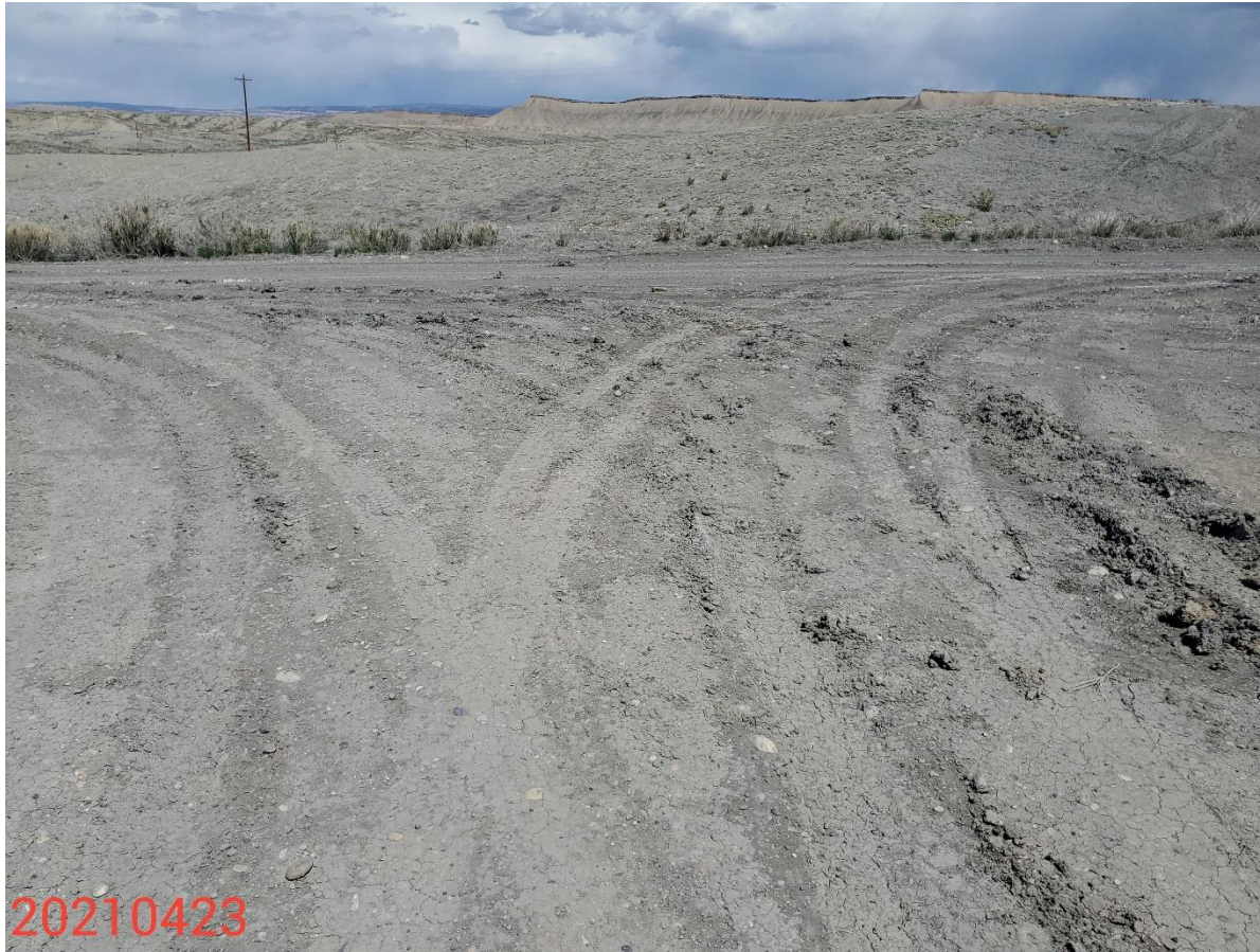
Photo 5 Photo taken from the access road entrance, facing north. Photo shows control measures to stabilize the production areas, and prevent off-site sediment transport during wet conditions are missing or insufficient.
