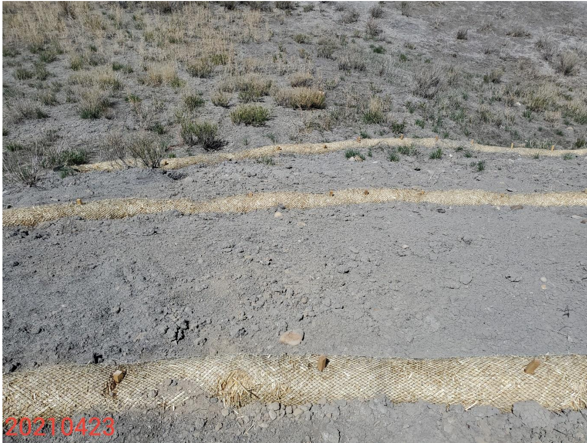
Photo 1: Photo taken from the west end of the Location. Photo shows that the gully erosion has been repaired, and control measures implemented.
