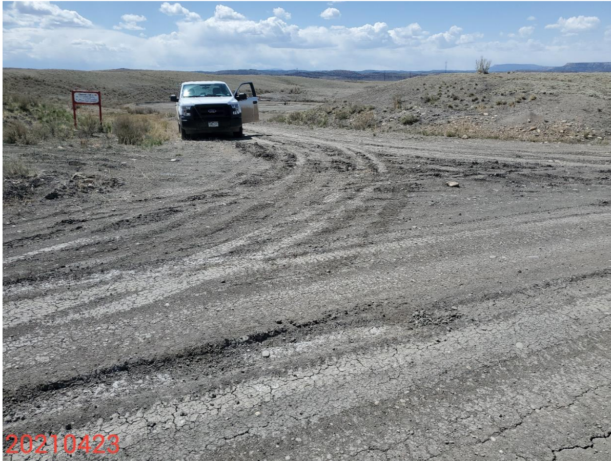
Photo 7: Photo taken from the access road entrance, facing south. Photo shows control measures to stabilize the production areas, and prevent off-site sediment transport during wet conditions are missing or insufficient.
