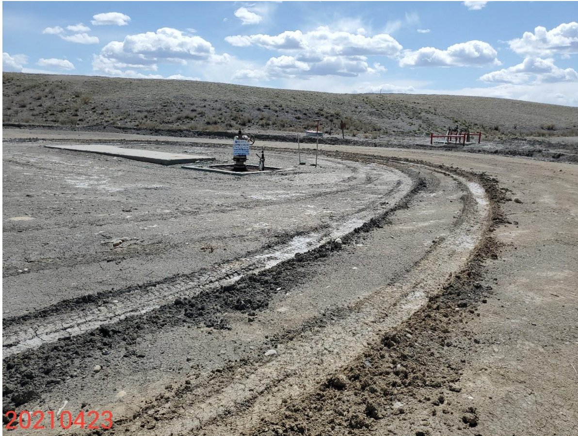
Photo 3: Photo taken from the west end of the production area, facing southeast. Photo shows control measures to stabilize the production areas, and prevent off-site sediment transport during wet conditions are missing or insufficient.
