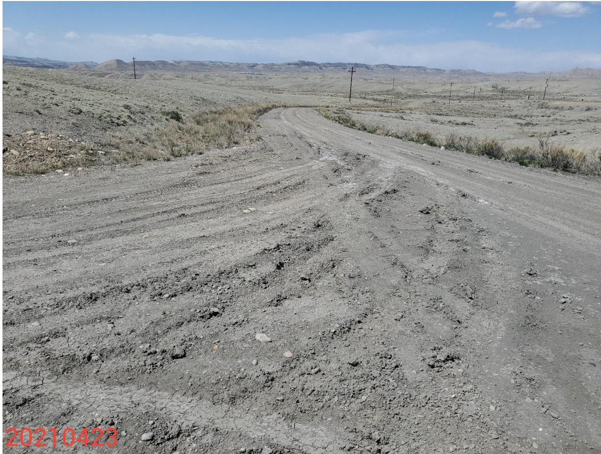
Photo 6: Photo taken from the access road entrance, facing west. Photo shows control measures to stabilize the production areas, and prevent off-site sediment transport during wet conditions are missing or insufficient.
