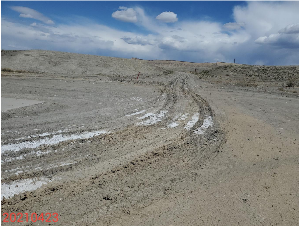
Photo 4: Photo taken from the southeast end of the production area, facing north. Photo shows control measures to stabilize the production areas, and prevent off-site sediment transport during wet conditions are missing or insufficient.
