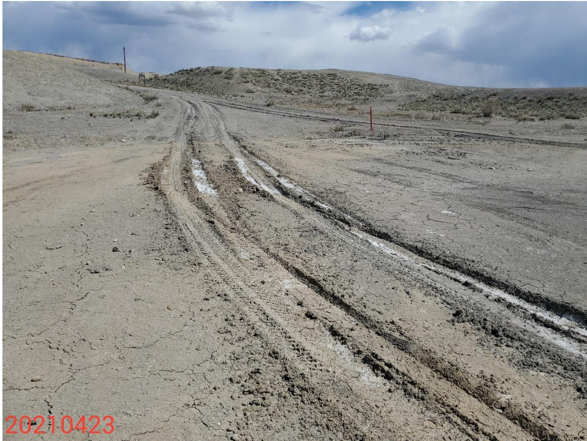
Photo 2: Photo taken from the west end of the production area, facing northeast. Photo shows control measures to stabilize the production areas, and prevent off-site sediment transport during wet conditions are missing or insufficient.
