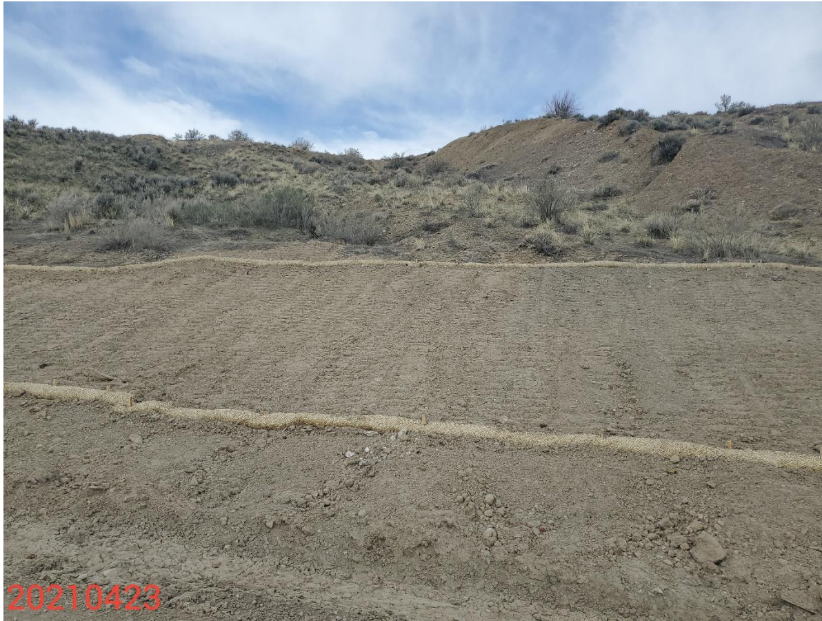
Photo 1: Photo taken from the Location, facing west. Photo shows slopes west of the road have been tracked, and wattles installed.
