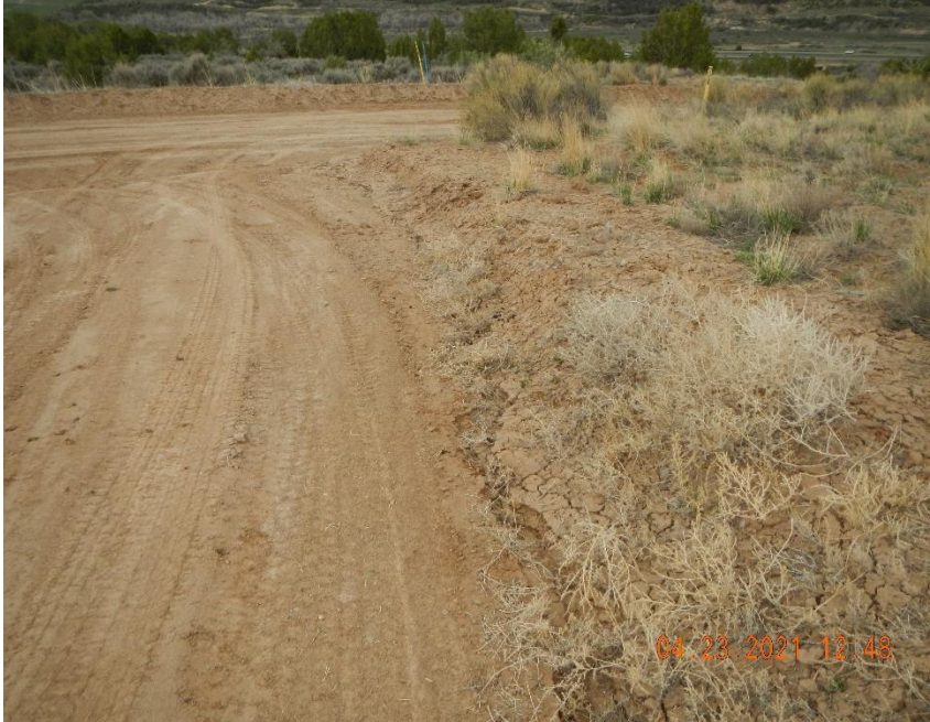
Soft sediment in ditch is riling.
