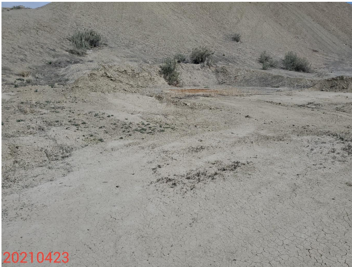
Photo 1: Photo taken from west end of the Location, facing north. Photo shows area where the tank was Location. Photo shows final reclamation activities including, but not limited to, compaction alleviation, recontouring/regrading and revegetation activities have not been conducted on Location and access road; photo also shows that the containment berm and area where tank was located remains evident.
