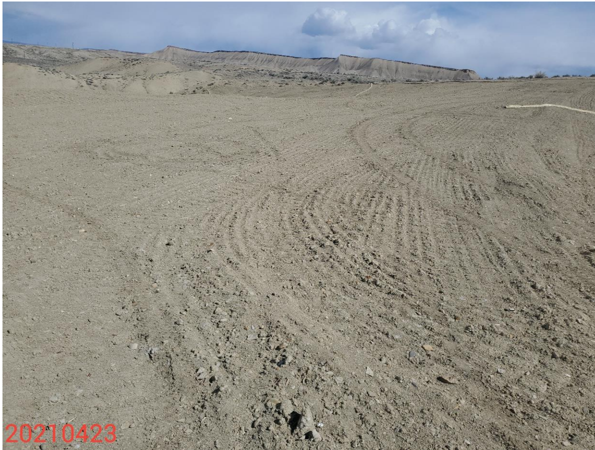
Photo 1: Photos 1-4 taken from the Location. Photos show additional erosion logs have been implemented on the Location. Operator does not appear to have implemented other BMPs in conjunction with erosion logs to stabilize the soils. Unclear if logs alone is sufficient to manage stormwater on Location.
