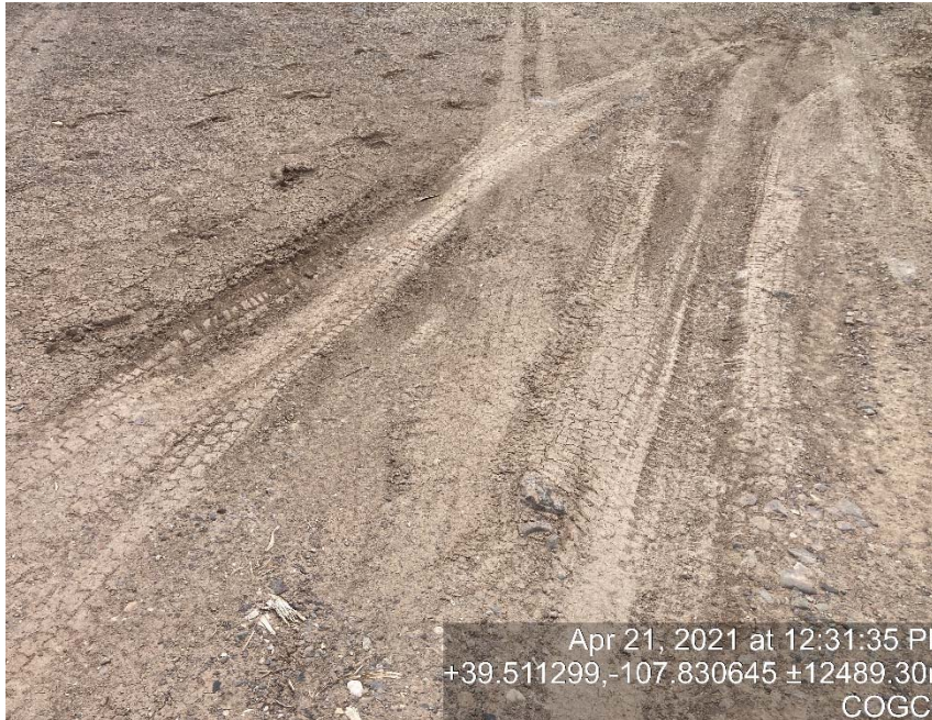
Lack of stabilization/compaction
