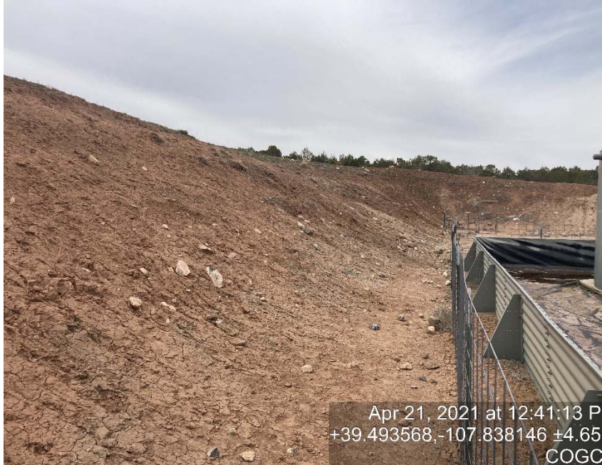
Lack of stabilization
