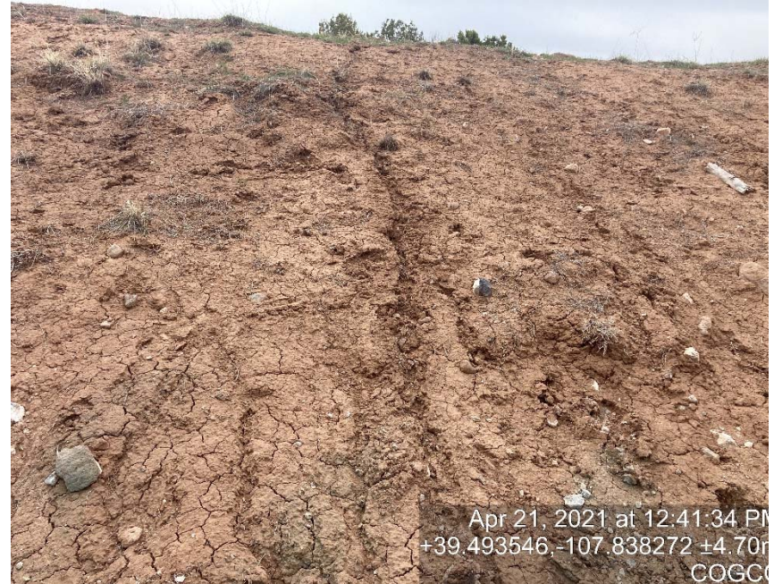
Lack of stabilization
