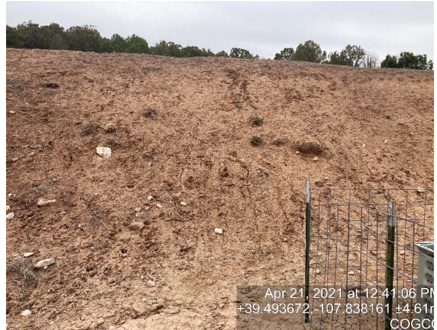
Lack of stabilization
