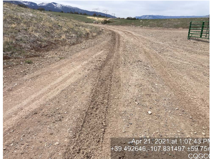
Lack of stabilization/compaction
