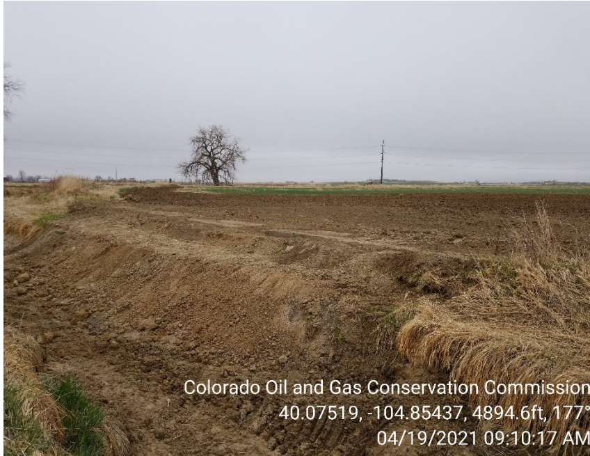
Photo 1 – Spill area. Excavation has been backfilled disturbed surfaces have been ripped.
