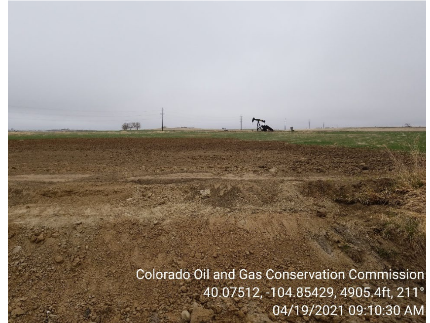
Photo 2 – Spill area. Excavation has been backfilled disturbed surfaces have been ripped.
