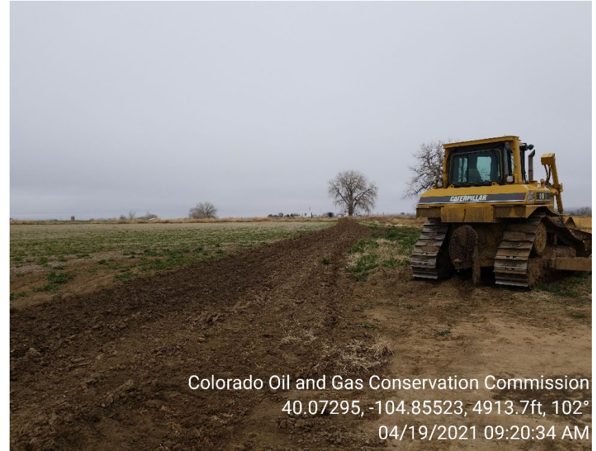
Photo 4 – Spill area access road; road has been ripped.
