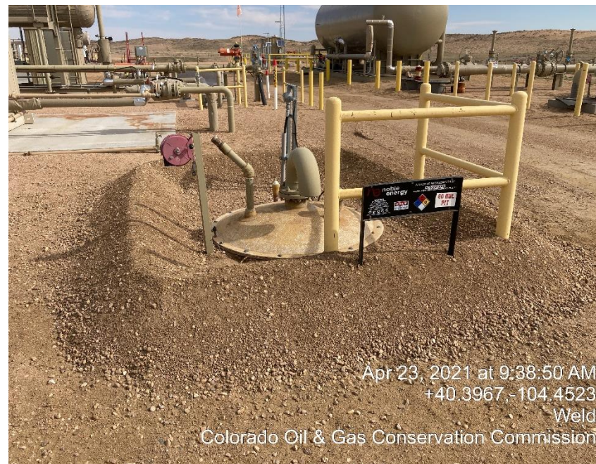
Photo #6 Repaired berm
