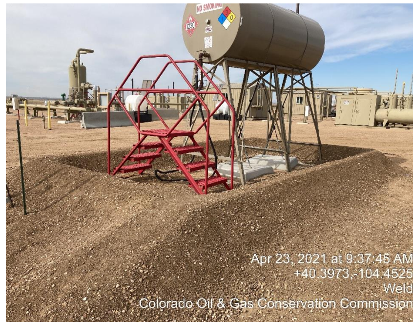
Photo #4 Repaired berm
